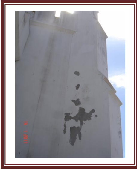
Fig. 9.1. Spalling on buttress.
