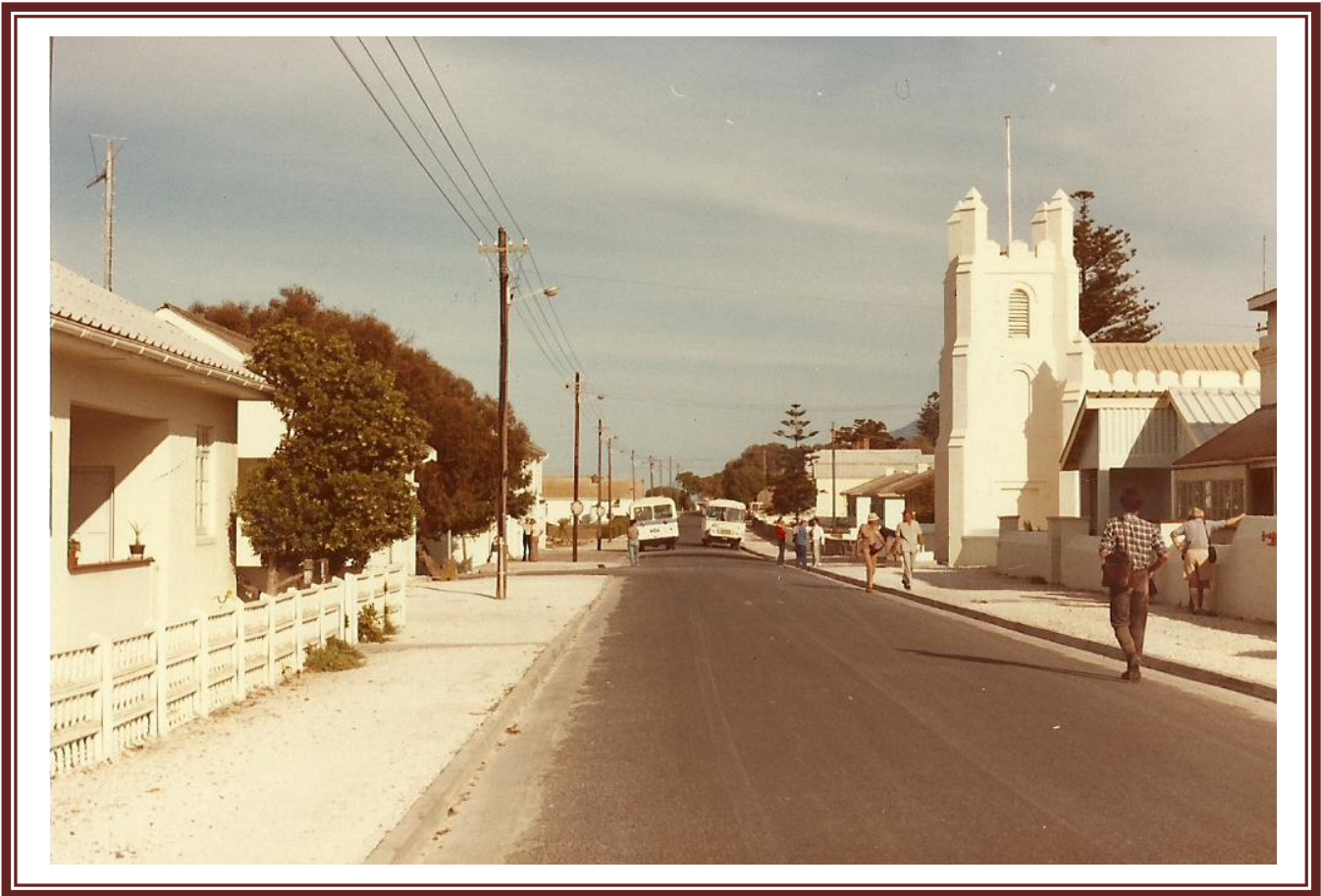
Fig. 7.3.4. Church streetscape ca 1983.
