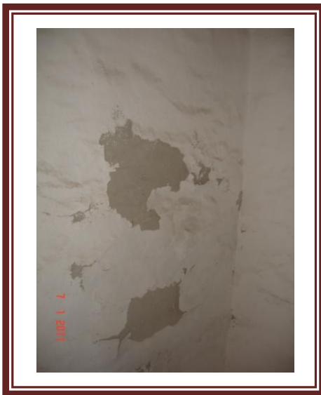
Fig. 9.4. Peeling paint inside tower.
