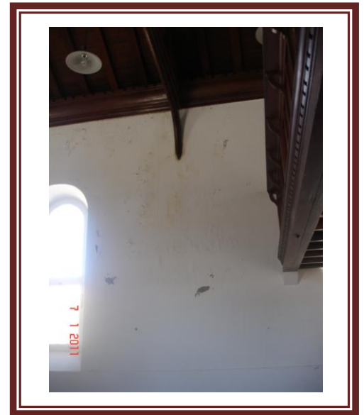
Fig.9.7. Interior water damage.
