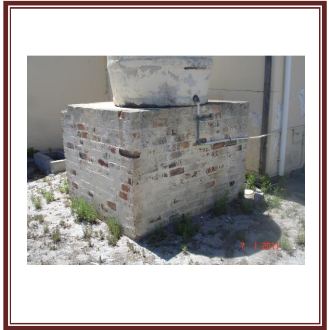
Fig.6.16. Asbestos water tank
