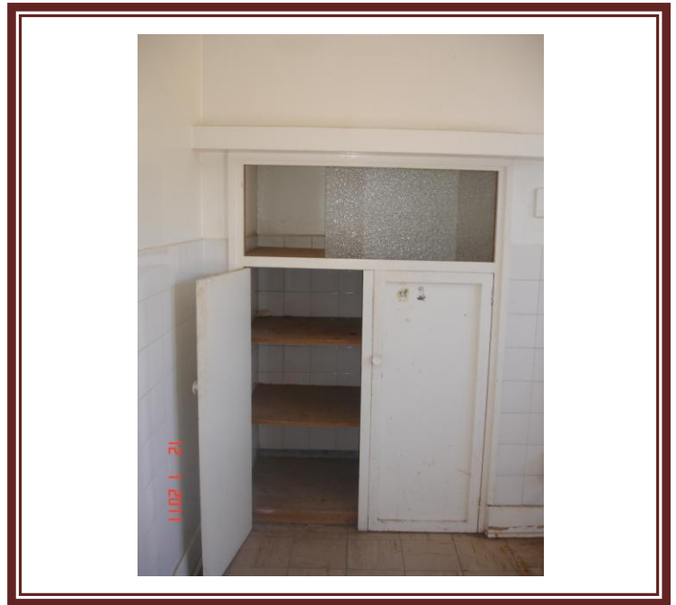
Fig.7.1.12 Alcove for coal stove in kitchen. Cupboard is later addition after removal of stove.
