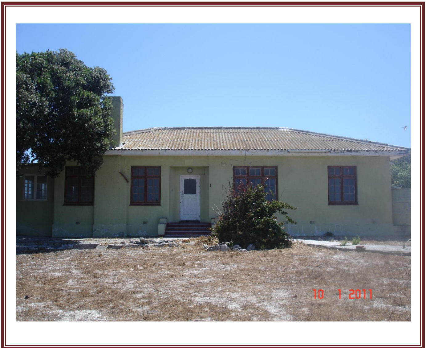
Fig.7.2.1. Front, facing east towards Table Mountain.
