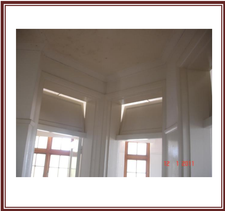
Fig.7.1.11. Doors with painted fanlights
