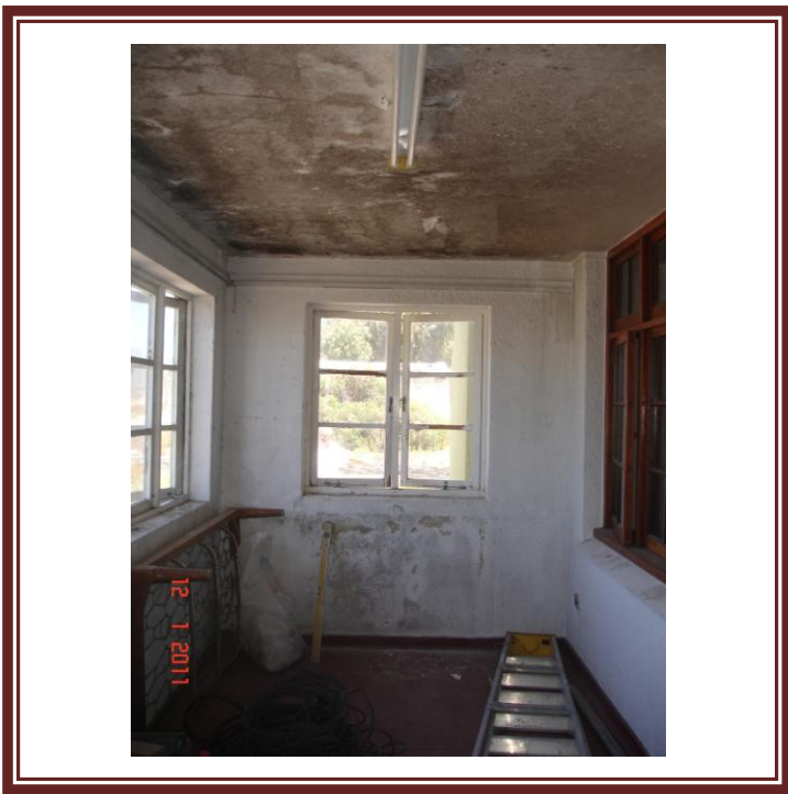
Fig.7.1.9. Interior of enclosed verandah
