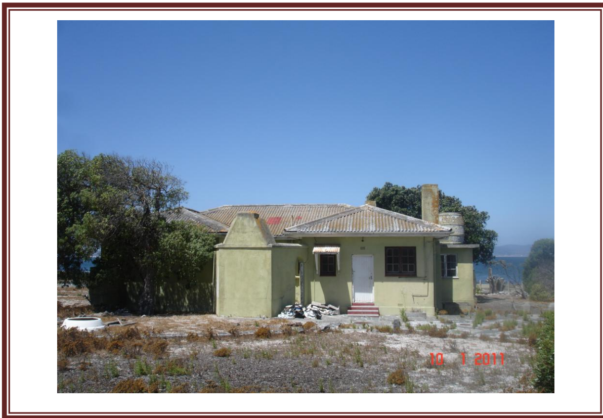
Fig.7.1.4. Rear facing west.
