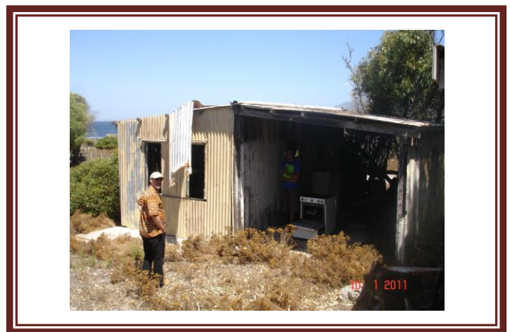
Fig.7.2.4. North face, garage original entrance clad with tin. Original wood exterior can be seen on inside of later tin extension.
