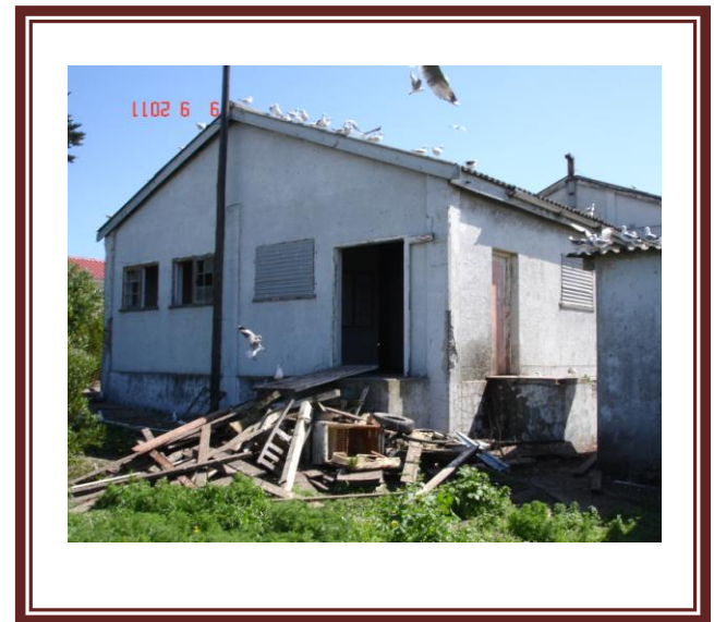
Fig.50. South wooden pole
