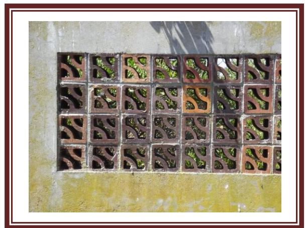
Fig.59. decorative ventilation interior east wall
