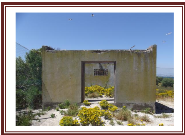
Fig.58. Entrance and west face
