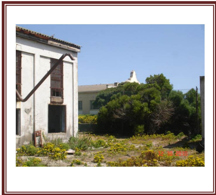
Fig.36. Stainless steel exhaust pipe
