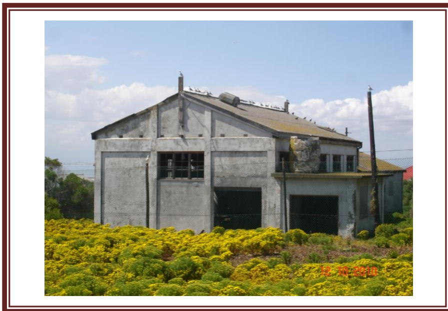
Fig.17. North gable wooden mounting. South gable siren mounting is discernable.
