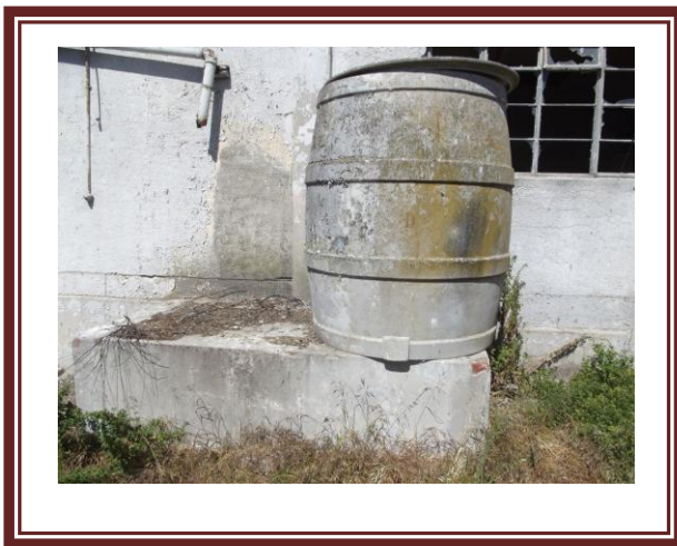
Fig.31. Left, East elevation tank
