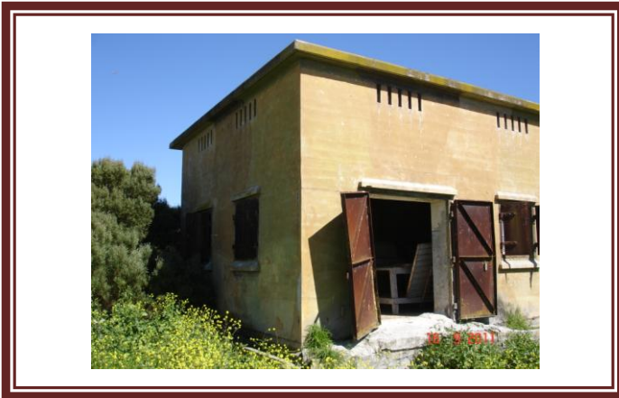
Fig.16. Entrance to Armory WWII ou Tronk
