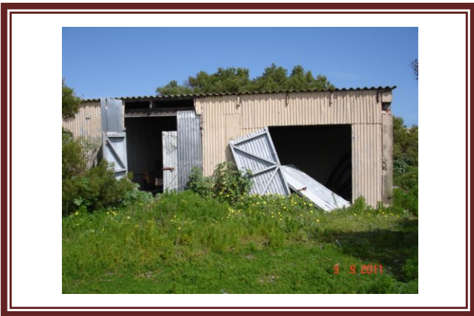
Fig. 18. Entrance to temporary storage
