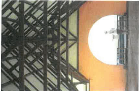
Timber kingpost-truss with "Mazista" shingle roof; Bagwash brickwork with horizontal pointing, painted.
