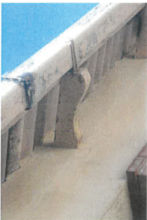
EAVES, SCALLOPED ENDS to Asbestos Fibre- cement gutters.
