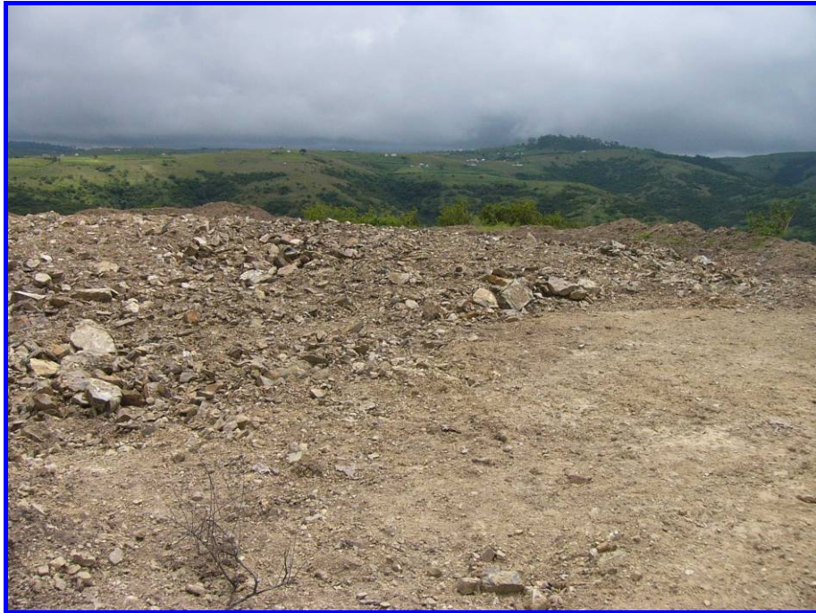
Figure 14: View of the existing borrow pit
