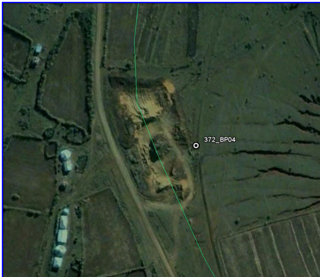
Figure 13: Aerial view - 372-BP04.
