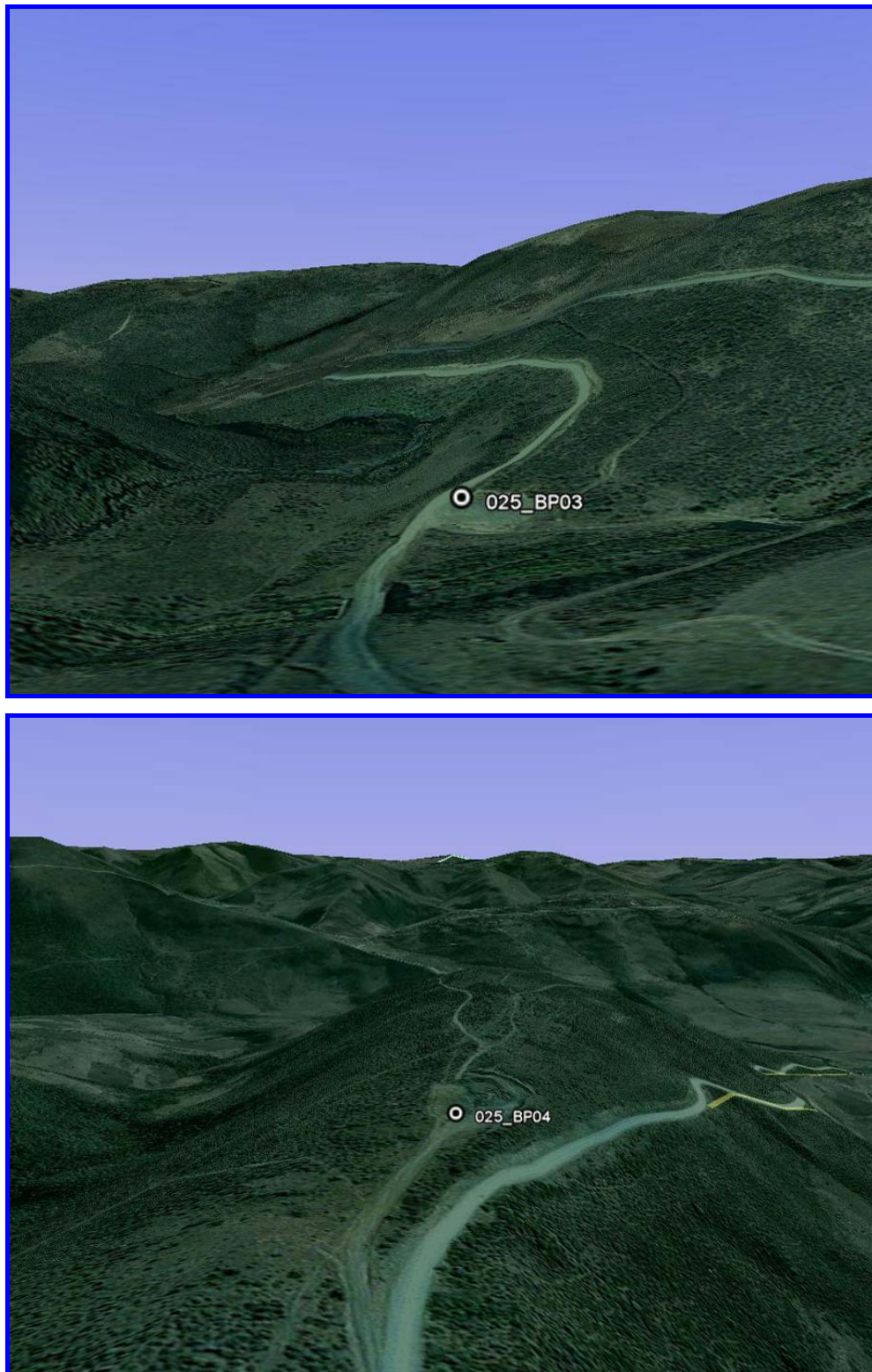
Figure 15: Terrain view indicating the position of the borrow pits in the landscape.
