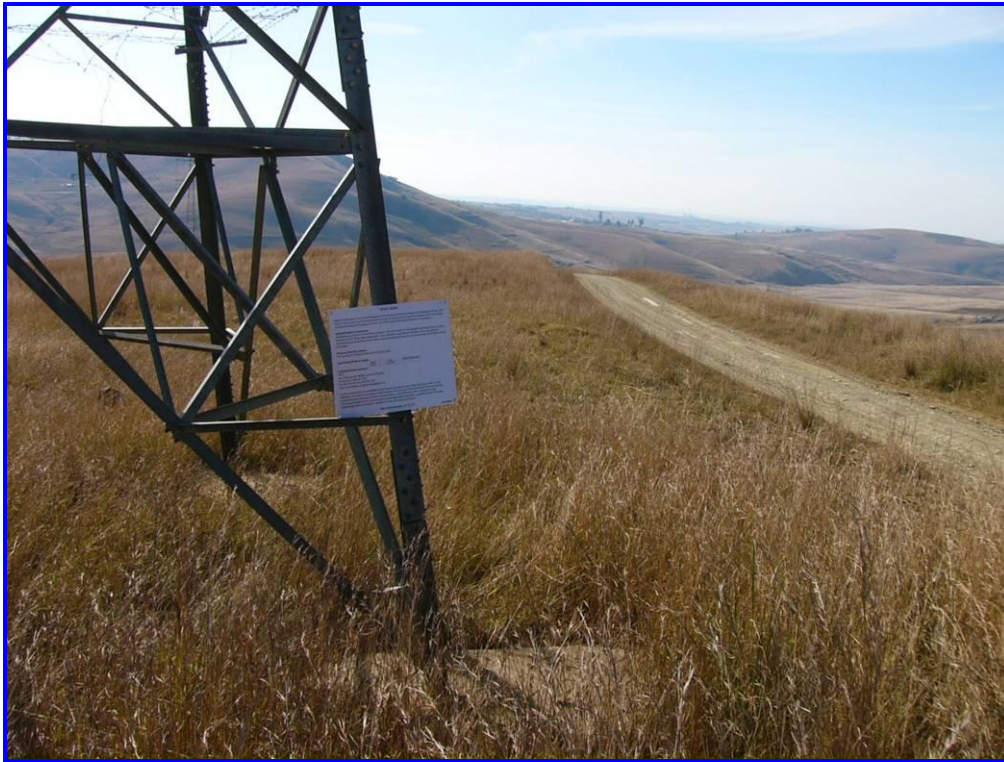
Figure 10: Images of the Signboards erected for DR08124.
