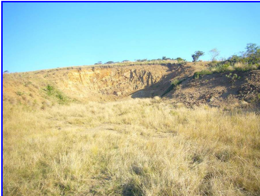
Figure 22: Borrow Pit # 151-BP04.
