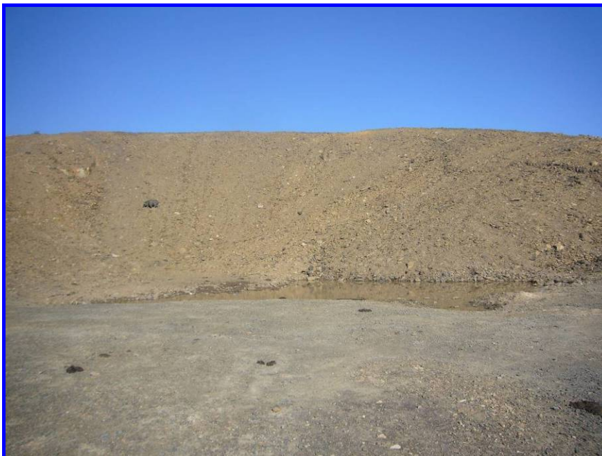
Figure 20: Borrow Pit # 151-BP02.
