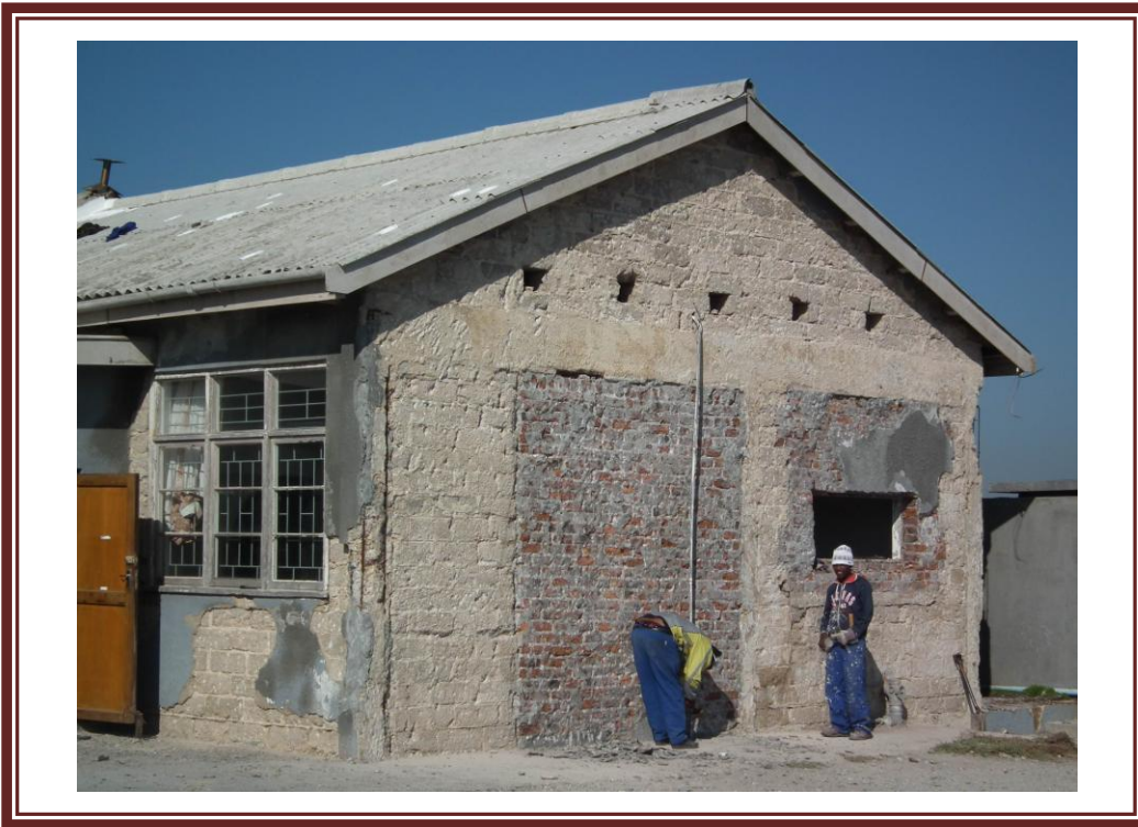
Fig.1. Features revealed after removal of plaster concur with earlier photographic and oral evidence.
