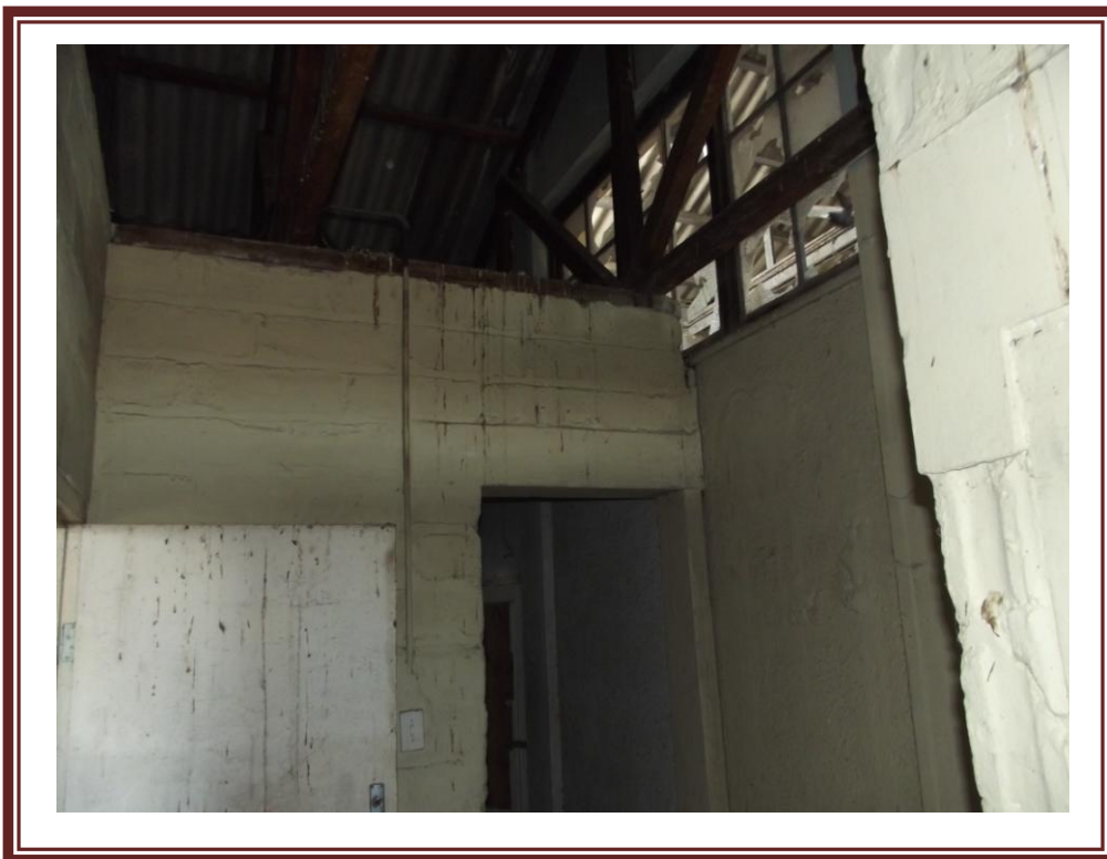
Fig.3. showing post supporting lintel.
