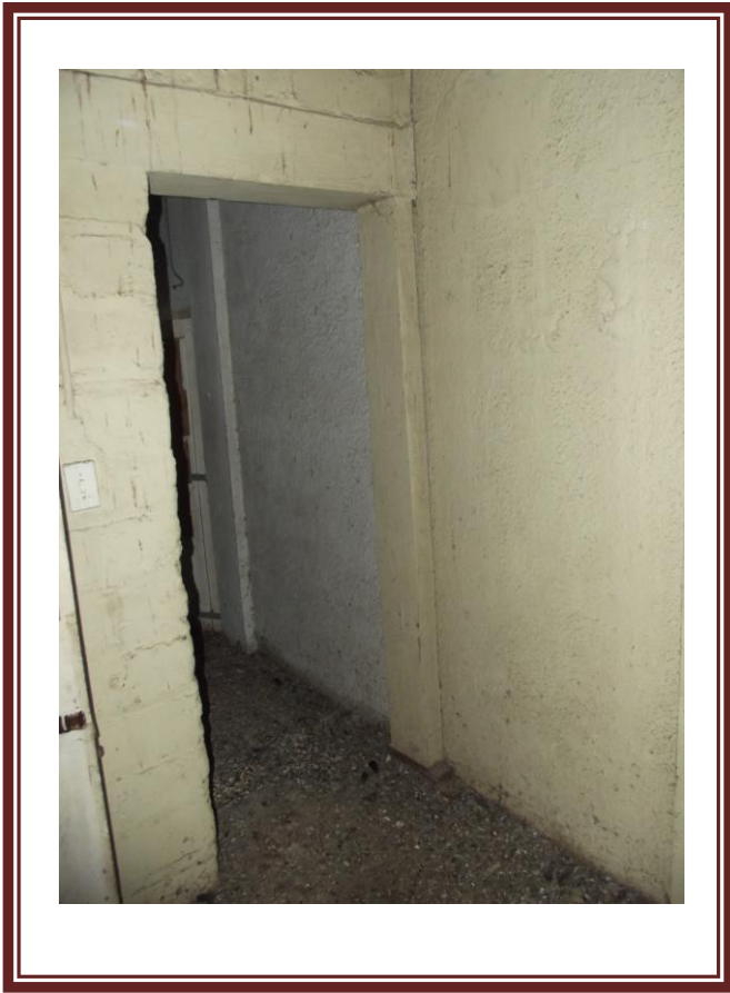
Fig. 1 & 2 showing wooden post supporting lintel.
