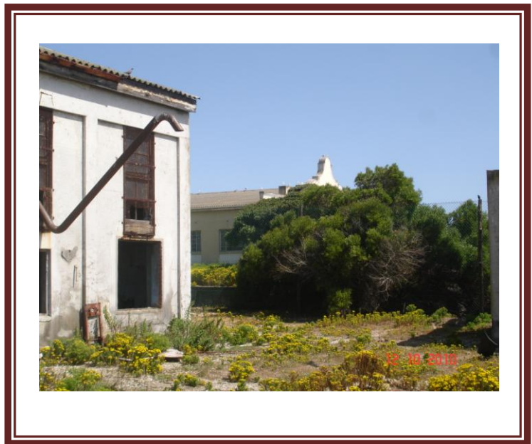
Fig.36. Stainless steel exhaust pipe
