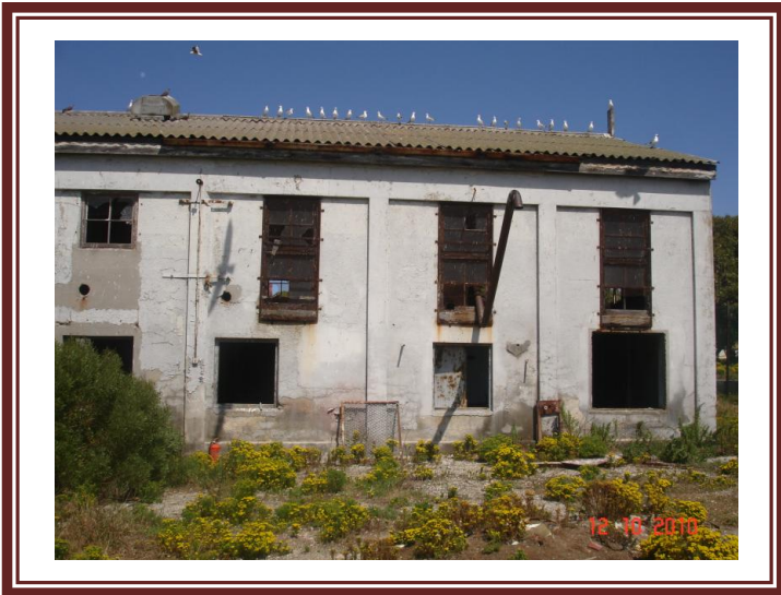
Fig.18. East elevation with extant section of steel guttering.
