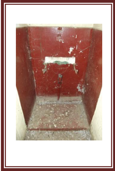
Fig.46. Left, Urinal and wash basin mounting
