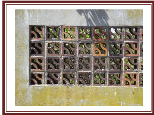
Fig.59. decorative ventilation interior east wall
