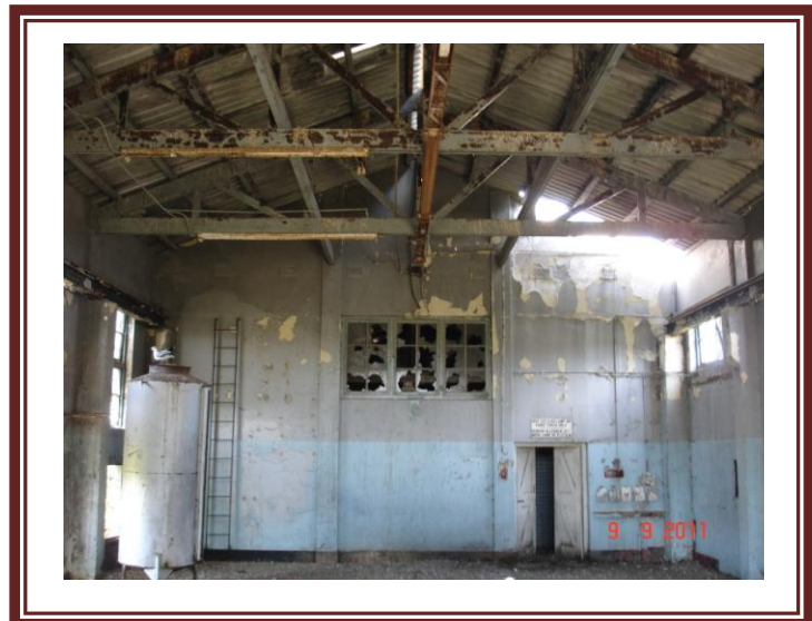
Fig.24. Steel ladder in SE corner and double wooden door opposite
