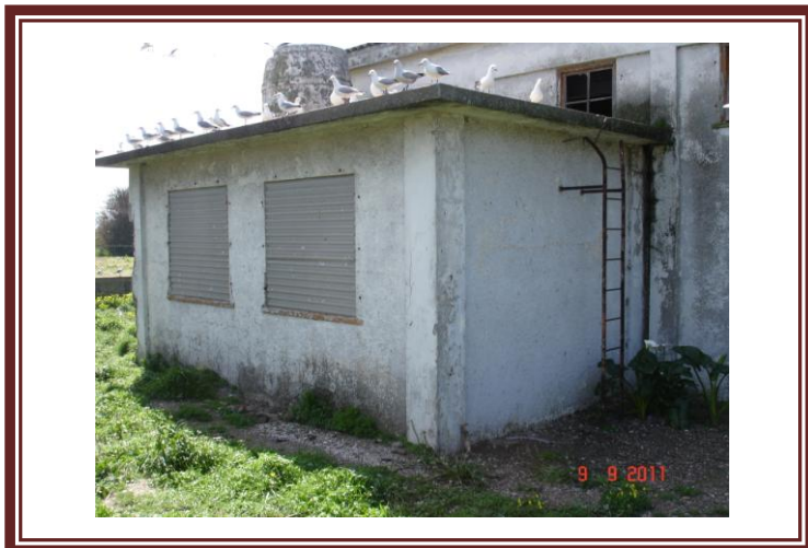
Fig.30. Steel ladder on South exterior wall
