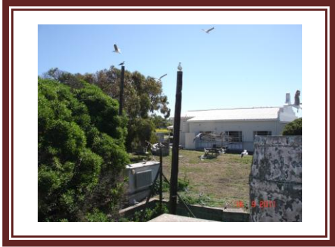
Fig.60 to 66. Fence , gate , retaining walls
