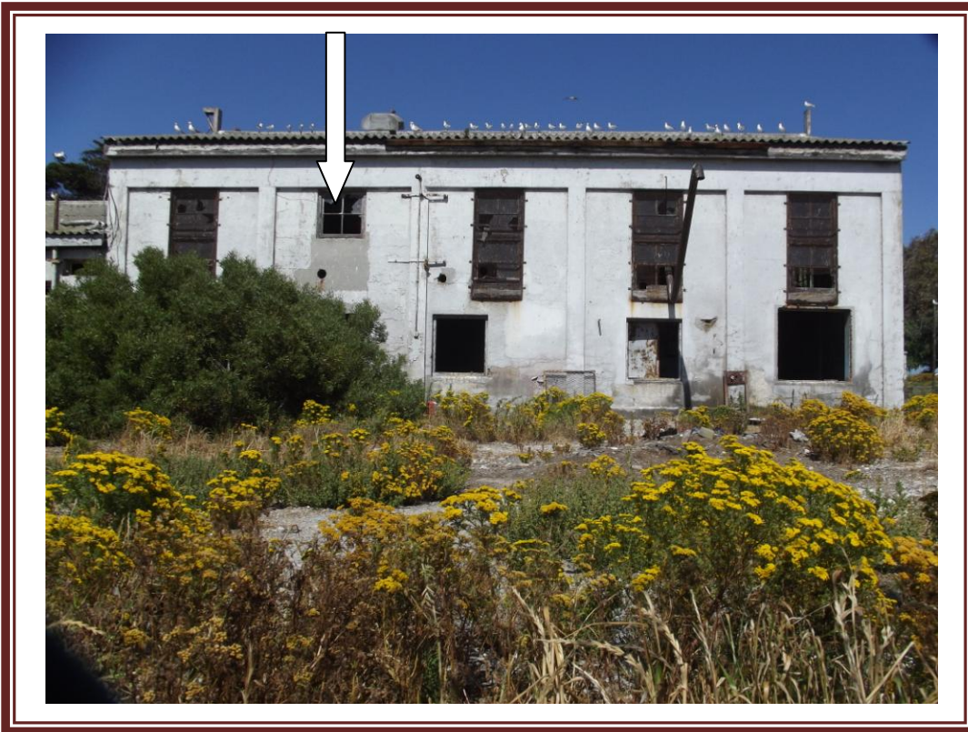
Fig. 7. Halved window of ca 1970's conversion in section B-C
