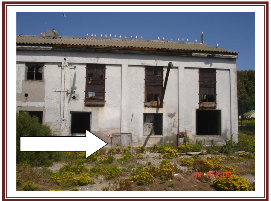
Fig.53. Remaining example of steel mesh grille
