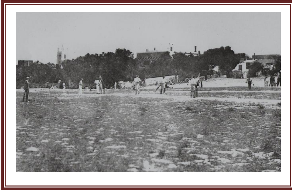
Fig. 11a. Ca 1920. The area where the OPS is now situated is parkland with large close knit trees
