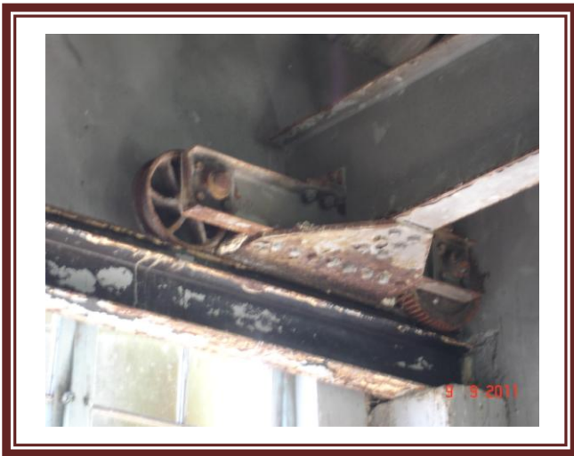
Fig. 20. Gantry with wheels on rail. SW corner of building left.
