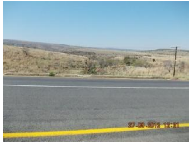
This picture shows culvert 4 over the Klip River Tributary looking East.
