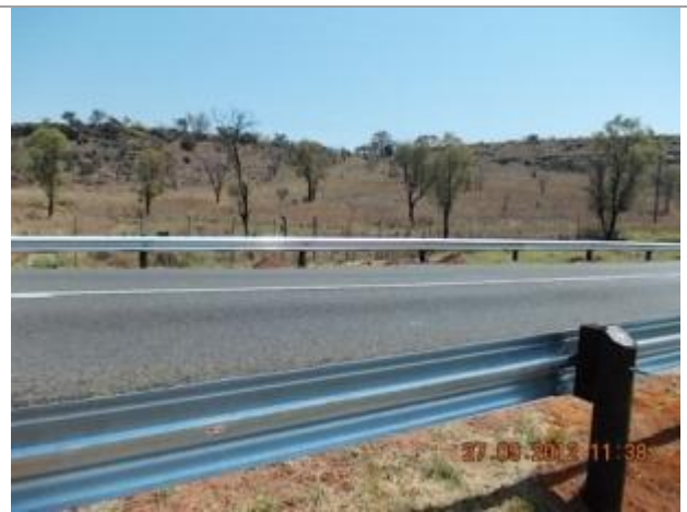
This picture shows culvert 2 over the Klip River Tributary looking West.
