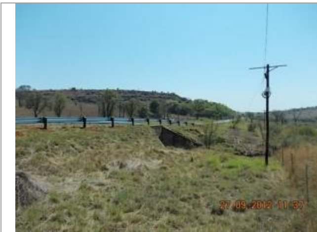
Picture depicting the existing N11 road between Middelburg and Loskop Dam. This picture shows culvert 2 over the Klip River Tributary looking Northwest.
