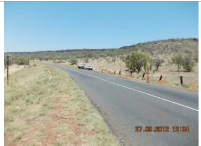
This picture shows culvert 3 over the Klip River Tributary looking South.
