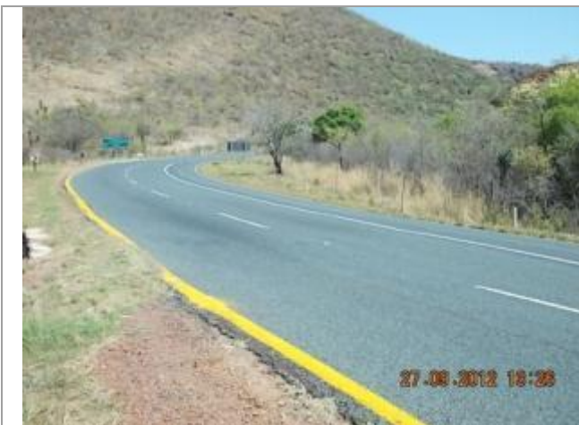
This picture shows culvert 5 over the Furrow looking Southwest.
