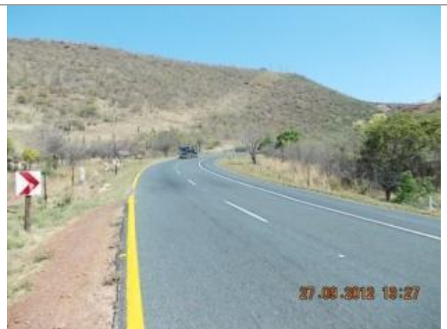
This picture shows culvert 5 over the Furrow looking South.
