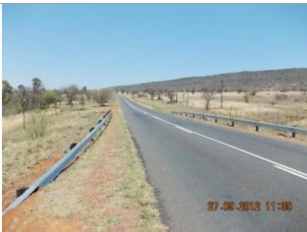
This picture shows culvert 2 over the Klip River Tributary looking South.
