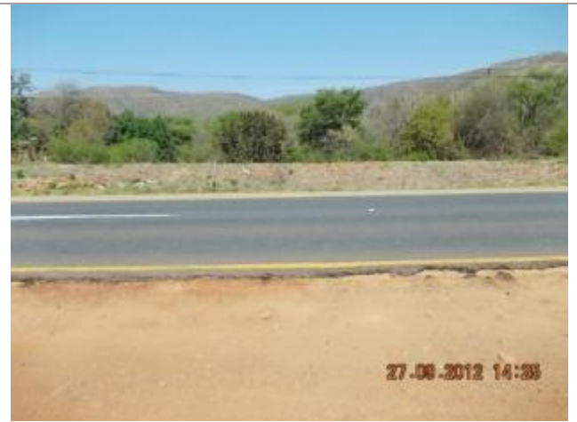
Picture depicting the existing N11 road between Middelburg and the Olifants River Bridge. This picture shows culvert 8 over the Olifants River Tributary looking East.
