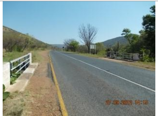
This picture shows Bridge 1749 over irrigation canal looking South.
