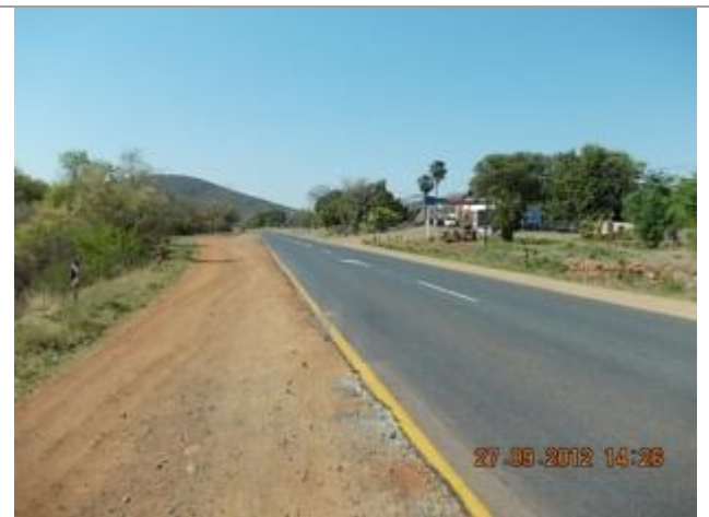
Picture showing culvert 8 looking North.
