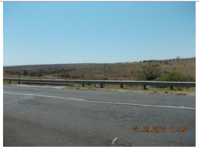
Picture depicting the existing N11 road between Middelburg and Loskop Dam. This picture shows Bridge B2136 over the Klip River Tributary looking East.
