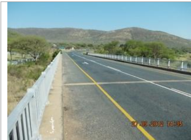
This picture shows Bridge 3611 over the Olifants River looking South.
