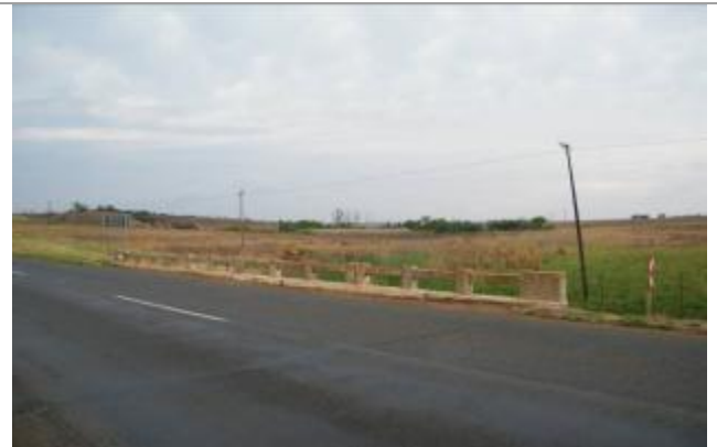
Picture showing the Keerom Spruit Brige taken when looking Northeast
