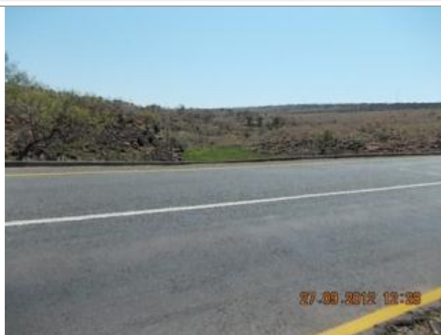
This picture shows culvert 4 over the Klip River Tributary looking West.
