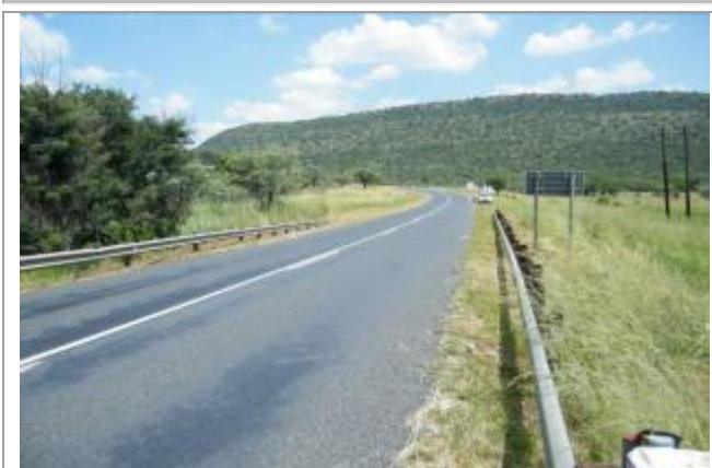
Picture taken from the existing Kranspoort River when looking South
