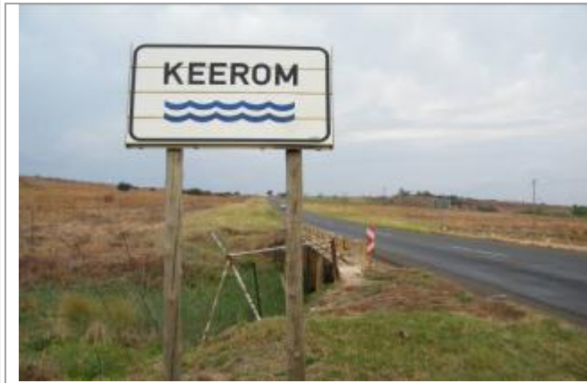
Picture showing the existing Keerom Spruit Bridge. This picture was taken looking North
