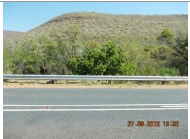
This picture shows culvert 7 over the Kranspoort Spruit Tributary looking South.
