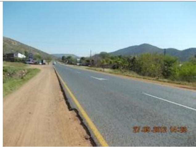
This picture shows culvert 8 over the Olifants River Tributary looking South.
