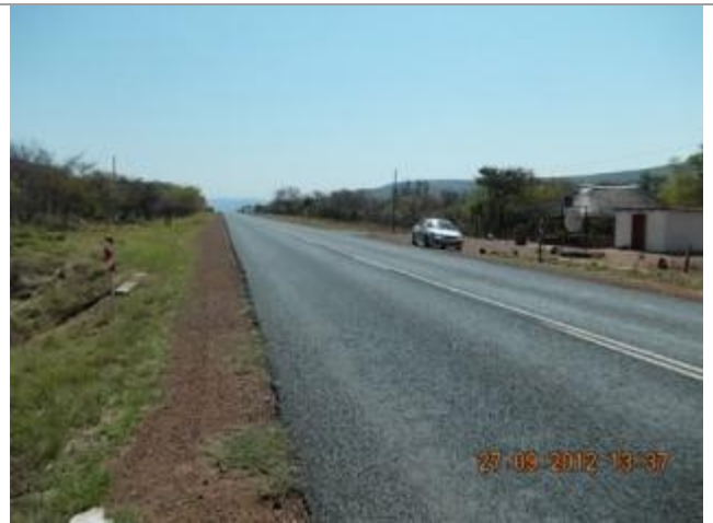
This picture shows culvert 6 over the Kranspoort Spruit Tributary looking West.
