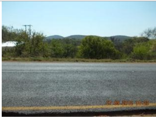
This picture shows culvert 8 over Olifants River Tributary looking West.
