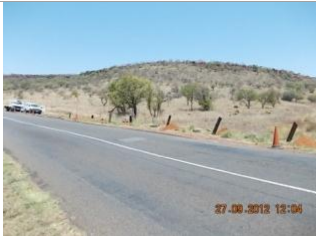
This picture shows culvert 3 over the Klip River Tributary looking Southwest.
