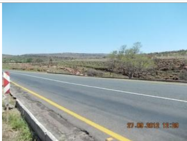
This picture shows culvert 4 over the Klip River Tributary looking Southwest.
