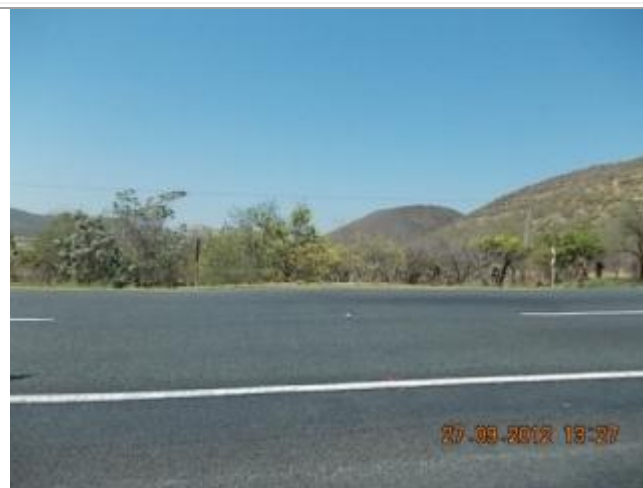
Picture depicting the existing N11 road between Middelburg and Loskop Dam. This picture shows culvert 5 over the Furrow looking East.
