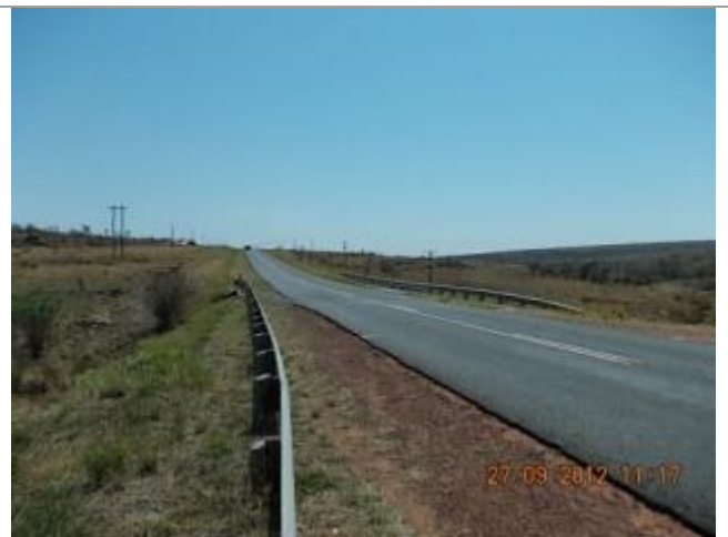
Picture showing Bridge B2136 over the Klip River Tributary looking North.
