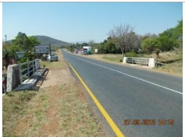
This picture shows Bridge 1749 over irrigation canal looking North.
