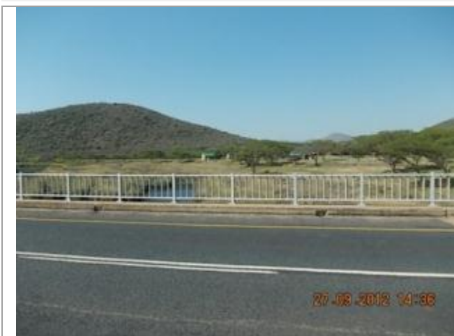
Picture depicting the existing N11 road between Middelburg and the Olifants River
