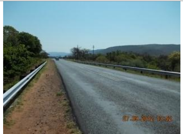
This picture shows culvert 7 over the Kranspoort Spruit Tributary looking West.
