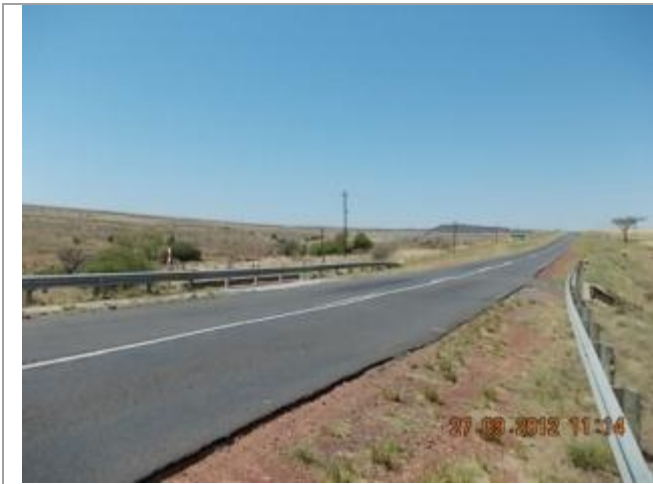
Picture depicting the existing N11 road between Middelburg and Loskop Dam. This picture shows Bridge B2136 over the Klip River Tributary looking Southeast.
