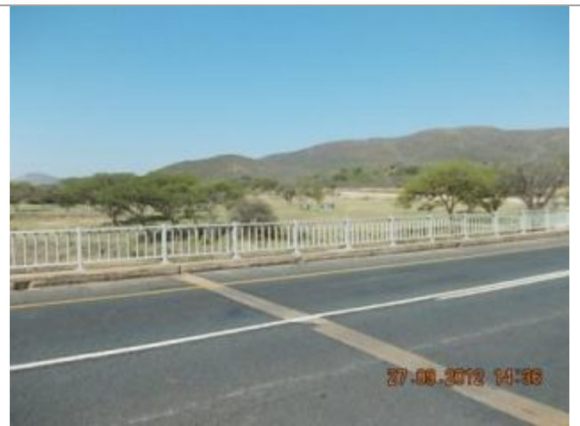
This picture shows Bridge 3611 over the Olifants River looking Southeast.
