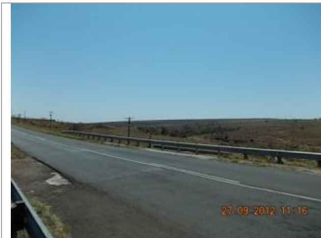
Picture showing Bridge B2136 across Klip River Tributary. This picture was taken looking Northeast.
