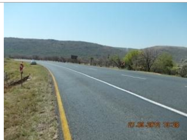
Picture showing culvert 5 looking North.
