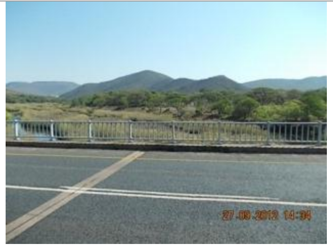
This picture shows Bridge 3611 over the Olifants River looking West.
