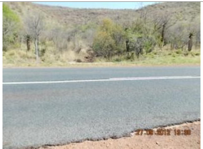
This picture shows culvert 6 over the Kranspoort Spruit Tributary looking South.
