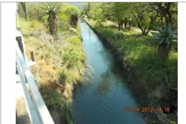
This picture shows the irrigation canal under Bridge 1749.
