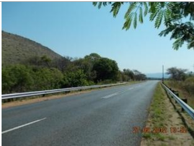
This picture shows culvert 7 over the Kranspoort Spruit Tributary looking Southwest.
