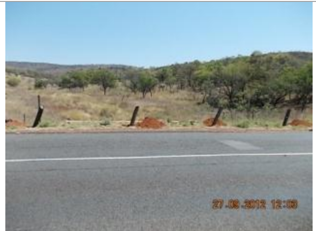
This picture shows culvert 3 over the Klip River Tributary looking West.
