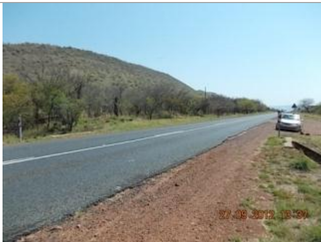
This picture shows culvert 6 over the Kranspoort Spruit Tributary looking Southwest.
