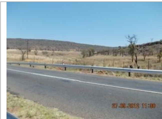
This picture shows culvert 2 over the Klip River Tributary looking Southwest.
