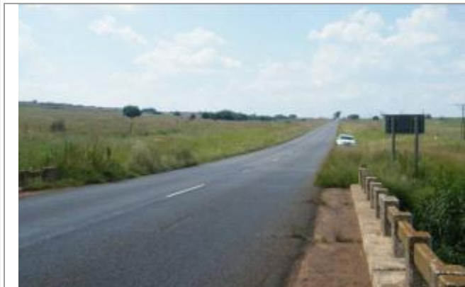
Picture showing the existing Keerom Spruit Bridge taken from the North.
