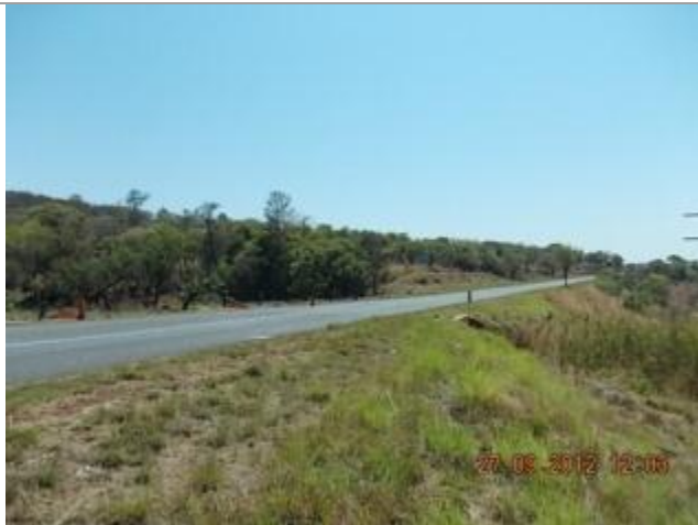
Picture depicting the existing N11 road between Middelburg and Loskop Dam. This picture shows culvert 3 over the Klip River Tributary looking Northwest.
