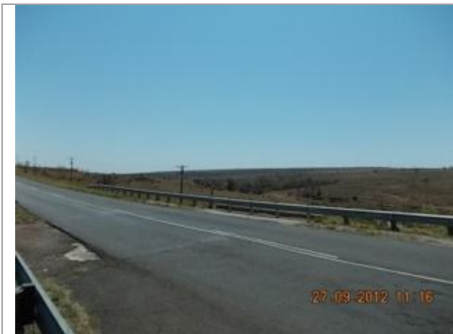
Picture showing culvert 2 across Klip River Tributary. This picture was taken looking Northeast.
