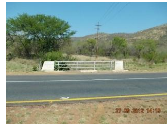
This picture shows Bridge 1749 over irrigation canal looking East.
