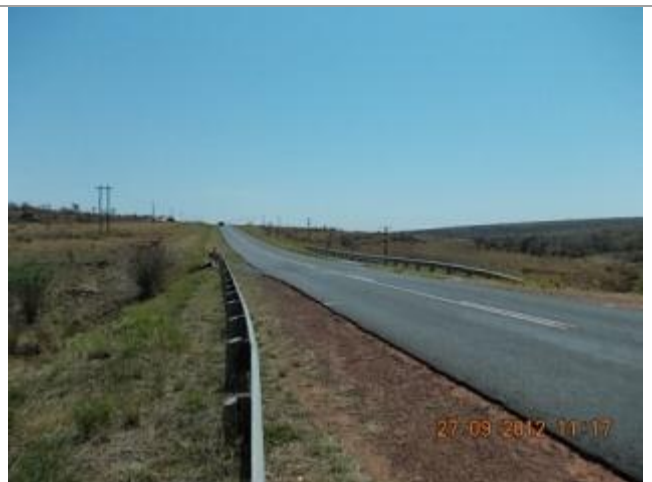
Picture showing culvert 2 looking North.
