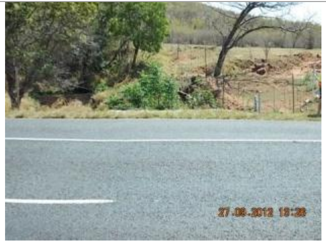
This picture shows culvert 5 over the Furrow Tributary looking West.
