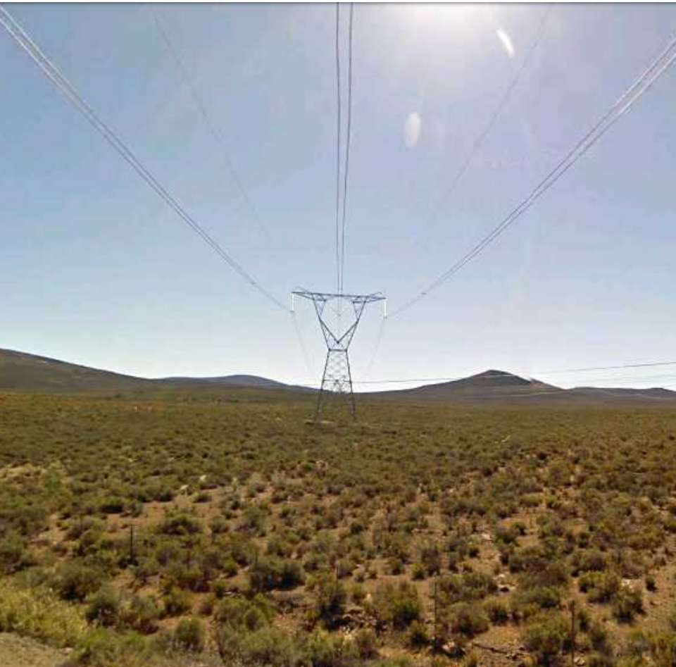
Southern 400kV power line
