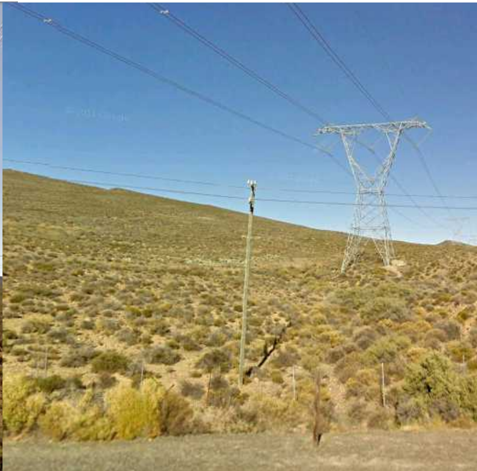
Northern 400kV power line
