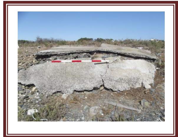
Fig.16. Collapsed west face
