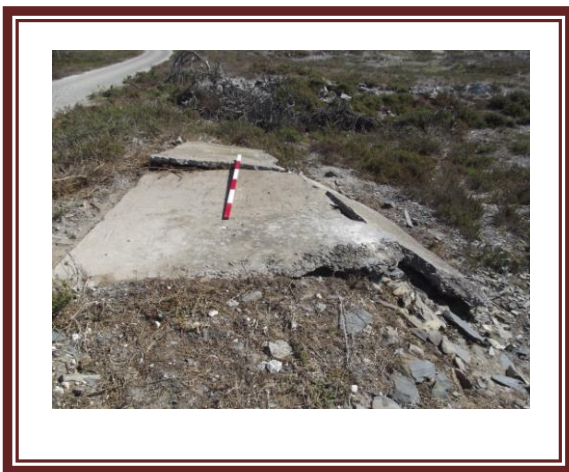
Fig.15. View towards south. Intact section
