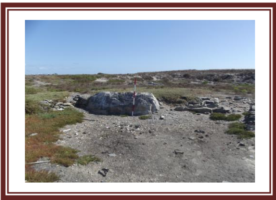
Fig.10. View of structure from North
