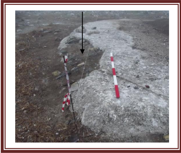
Fig.6. Eastern edge looking from N to S showing damaged section
