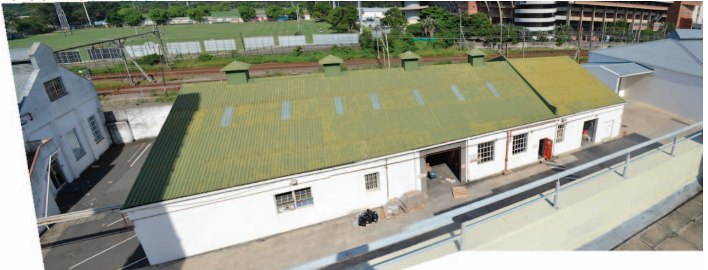
zone 04 | aerial view
