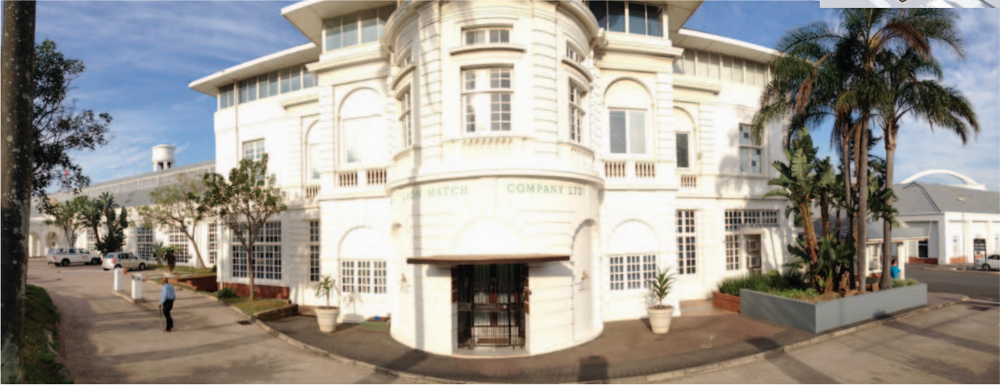
zone 01 | western facade and main entrance
