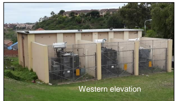
Photograph 1-Western elevation of sub-station building
