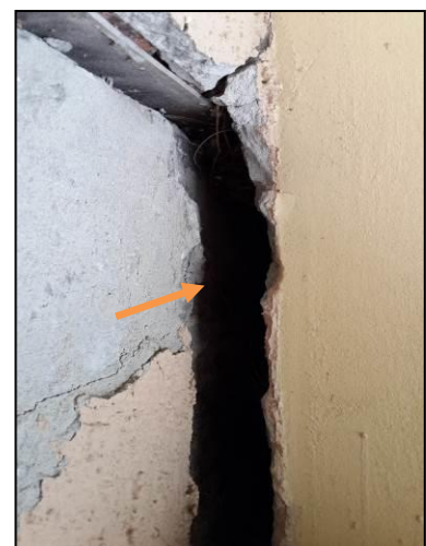
Photograph 5- Note 75 mm movement
