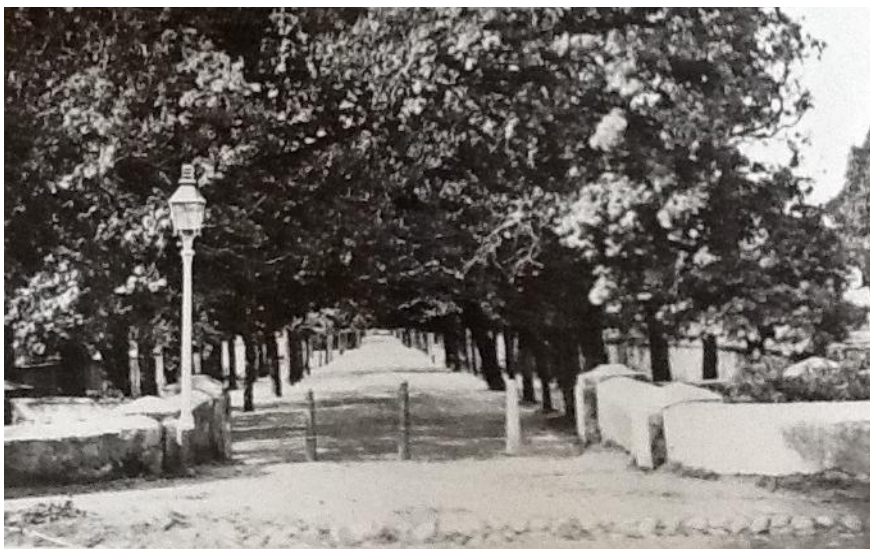
Figure 55: Entrance to Government Avenue, Cape Town from Orange Street. National Archives AG 1894.
