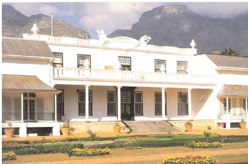
Figure 5: A contemporary view of the Tuynhuys (Bulpin 2003:31)
