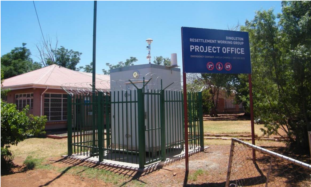
Figure 20: Dingleton PM 10 Monitoring station
