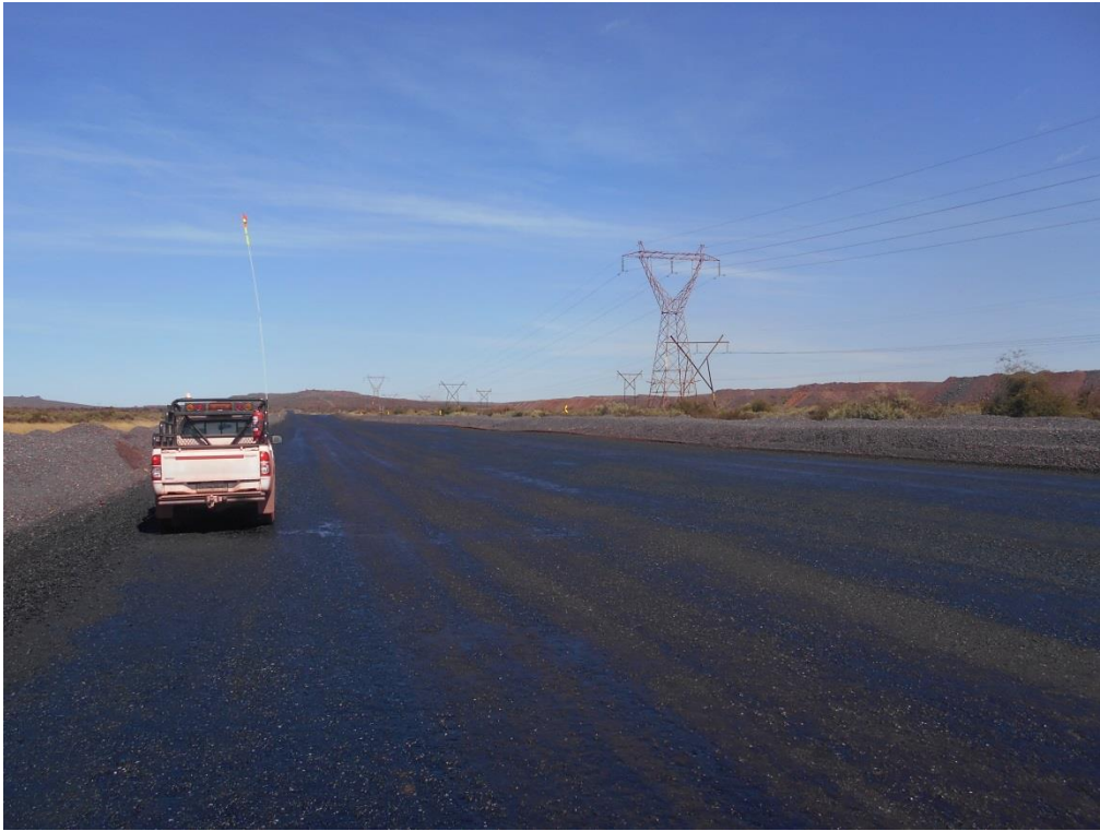
Figure 5: Current Lylyveld North haul road(treated with Dust-A-Side).
