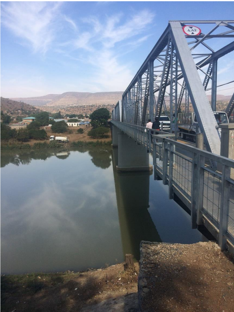
Figure 4: Upstream northern bank of existing bridge.
