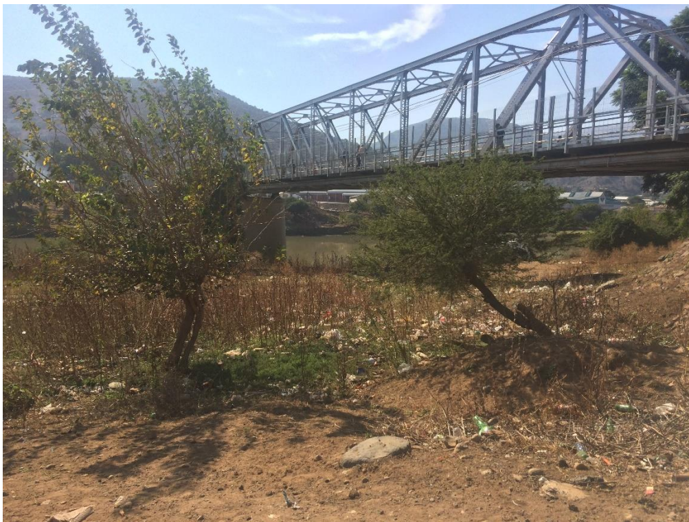
Figure 2: Downstream of existing bridge.
