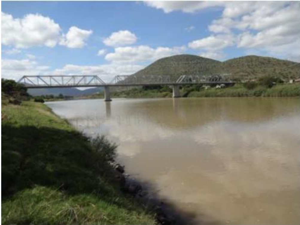
Figure 1: The existing one lane bridge at Tugela Ferry
