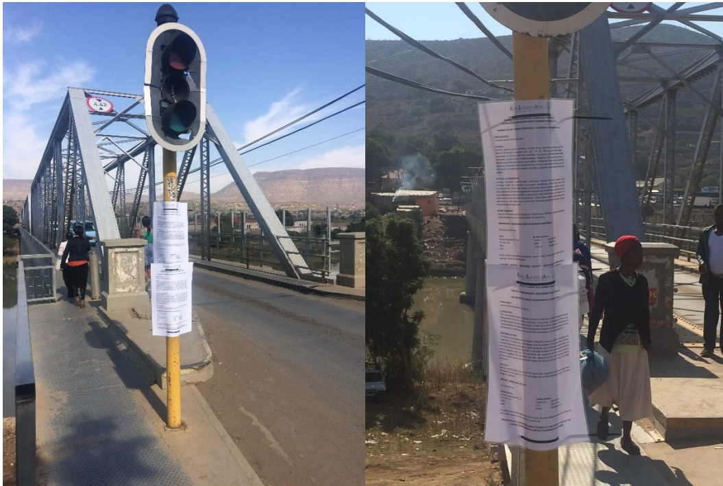
Figure 8 & 9: Notification displayed on the existing bridge (North and South).
