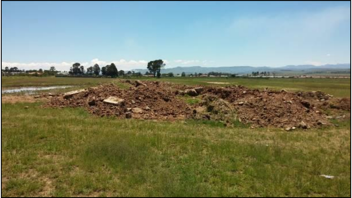
Figure 11: Soil excavation and soil/rubble dumping
