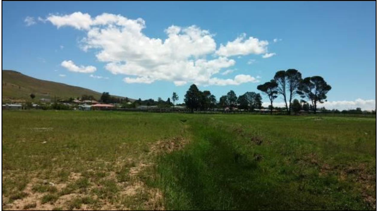
Figure 7: Stormwater drainage channel
