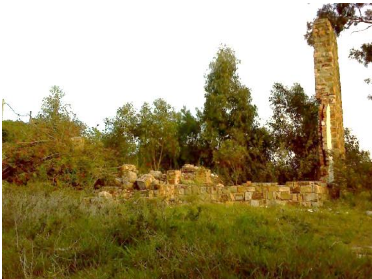
Figure 6: View of QBE3 with remains of foundations and chimney. Source: Celeste Booth, 2014.
