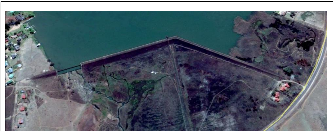
The dam wall (Photo: Google Earth)
