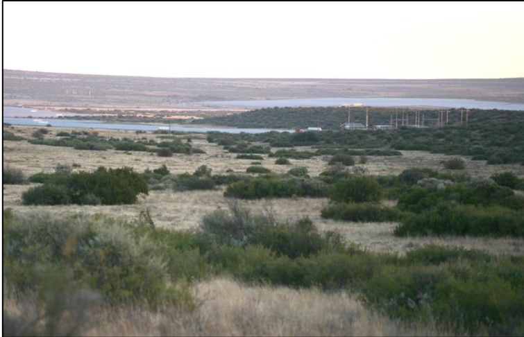
Looking towards the Jasper PV facility substation along the Redstone – Olien power line route. The rocky hills are dominated by Searsia ciliata with occasional Searsia lancea and Olea europea subsp. africana .
