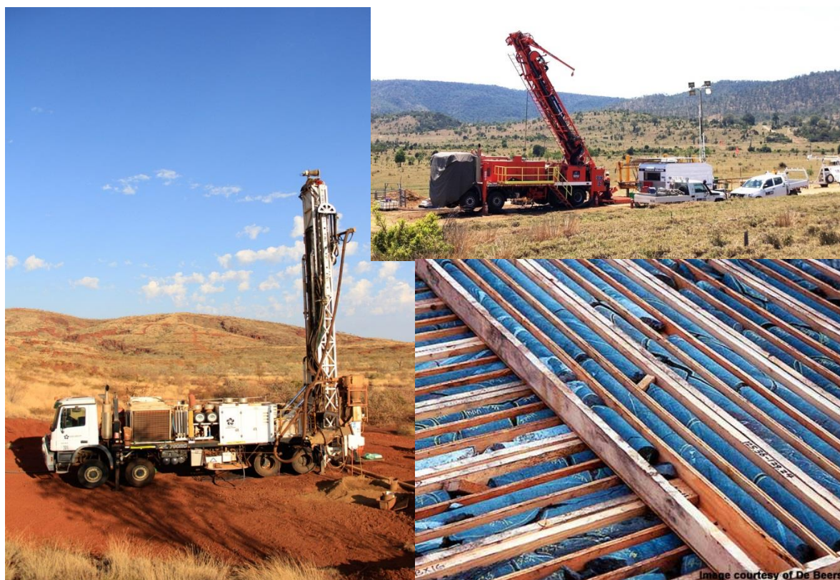
FIGURE 4-3: TYPICAL CORE BOREHOLE EQUIPMENT (Sources De Beers and Pinnacle Drilling)
