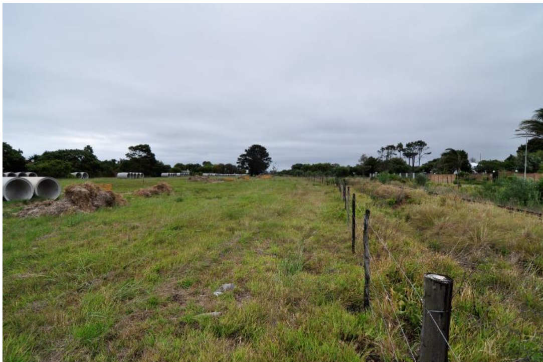
Plate 5: A view towards the Lorraine Substation with the small channel used to direct water away from the rail line visible along the right side of the fence. The area to the left of the is currently being prepared for the Lorraine stormwater pipeline
