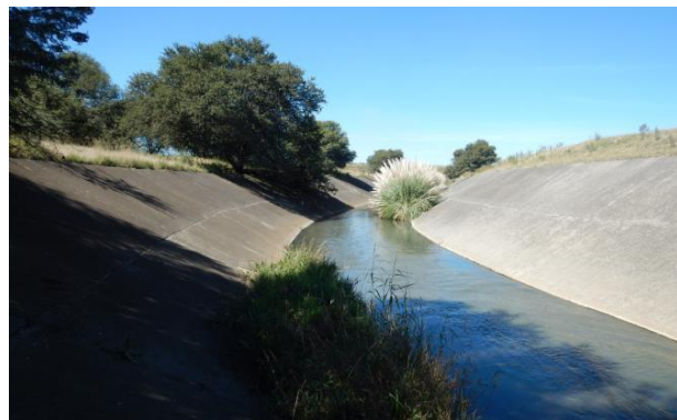
Concrete lined Vaal tributary downstream of the confluence
