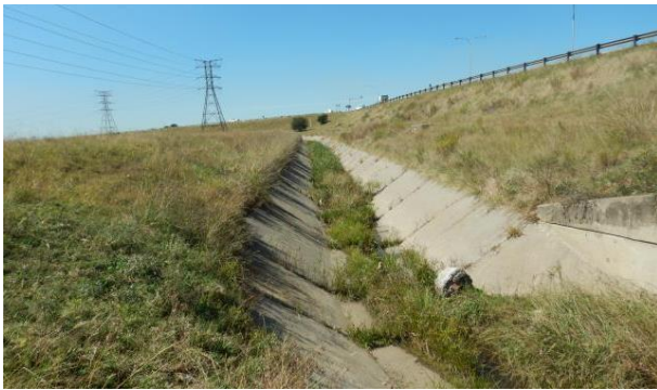
R28 drainage channel close to the confluence with R59 drainage channel
