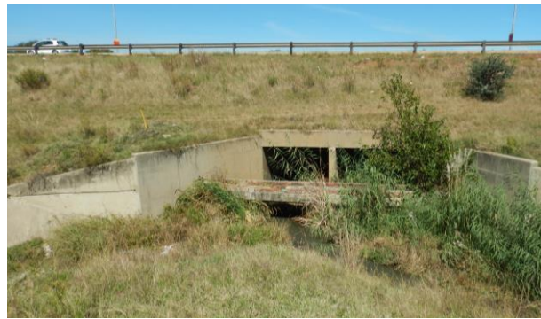
Culvert underneath the R28 Road
