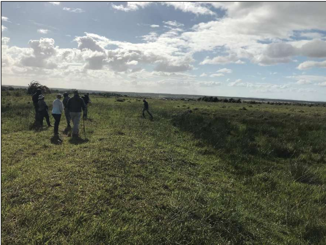
Figure 1.3 Photographic evidence of road interrupting natural flows in wetland. Area to the right of the road is the hillslope seep and area to the left (outside frame) is the bowl shaped wetland area.
