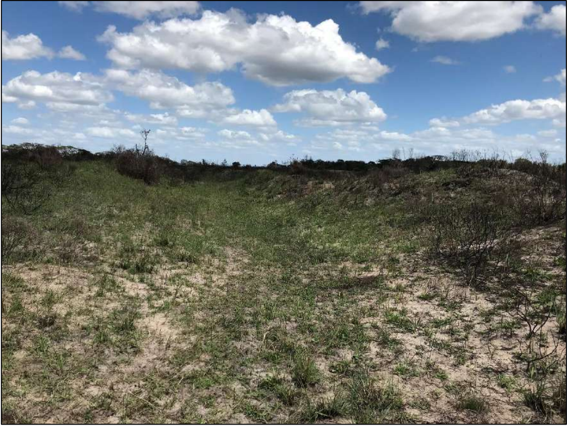
Figure 1.17 Photographic evidence of the excavated drain and the spoil deposits running along either side of the drain.
