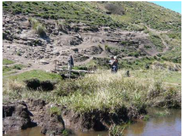
One of the cattle crossing places and the informal "bridge" that will be replaced by formal structures for both livestock and pedestrians
