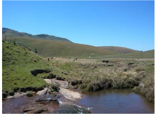
View down the lower reaches of the wetland towards Kolomane 16. Erosion of the channel at this point has taken place down to bedrock
