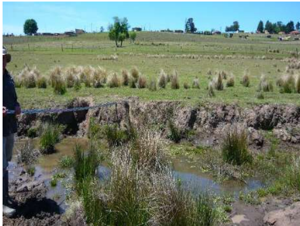
One of the drains that will be deactivated in the channel that has avulsed.
