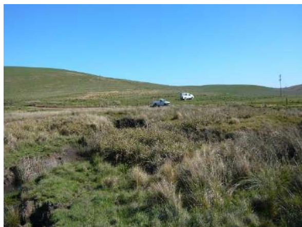
Looking across part of the toe of the wetland towards one of the headcut features to be stabilised (visible below the vehicles in the photograph)
