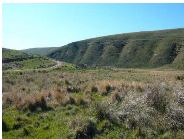
View from the toe of the wetland looking downstream. The gravel road that crosses the wetland is evident to the left
