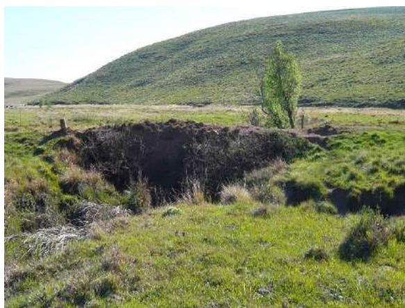
View from the toe of the wetland looking upstream across the gravel road and towards Kolomane 5. The eroded area is at the discharge point of the culverts that run under the road
