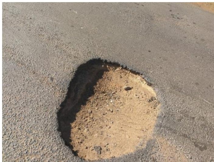
Photo 8: Potholing between Maple Street - EP Malan Street
