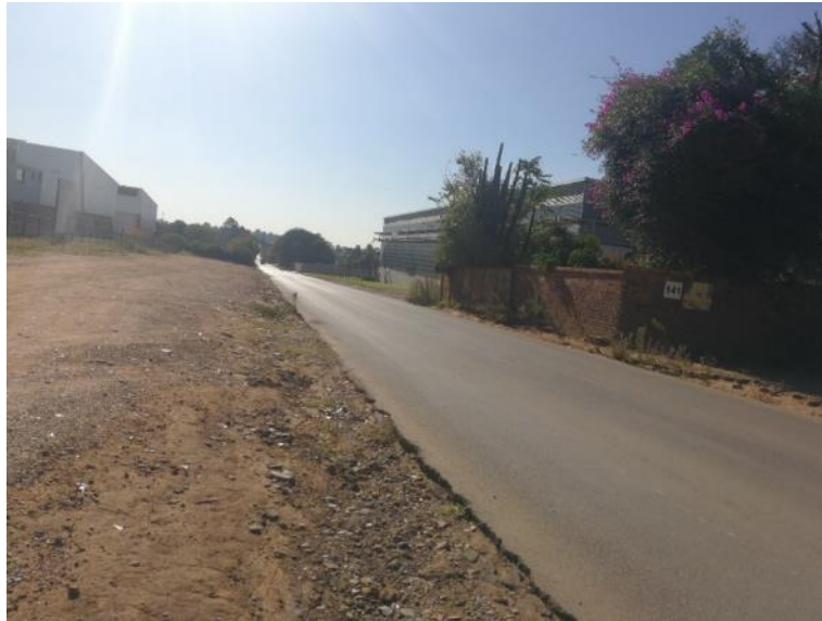
Photo 23: Road prism between Elgin Street and Deodar Street
