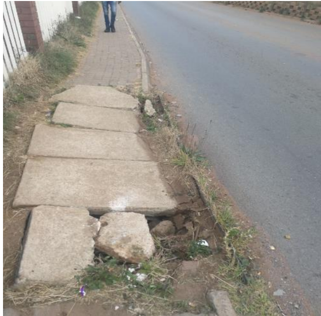
Photo 17: Blocked kerb inlet between Pomona Road - Maple Street
