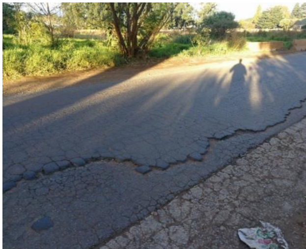
Photo 4: Advanced crocodile cracking between EP Malan Street - Elgin Street
