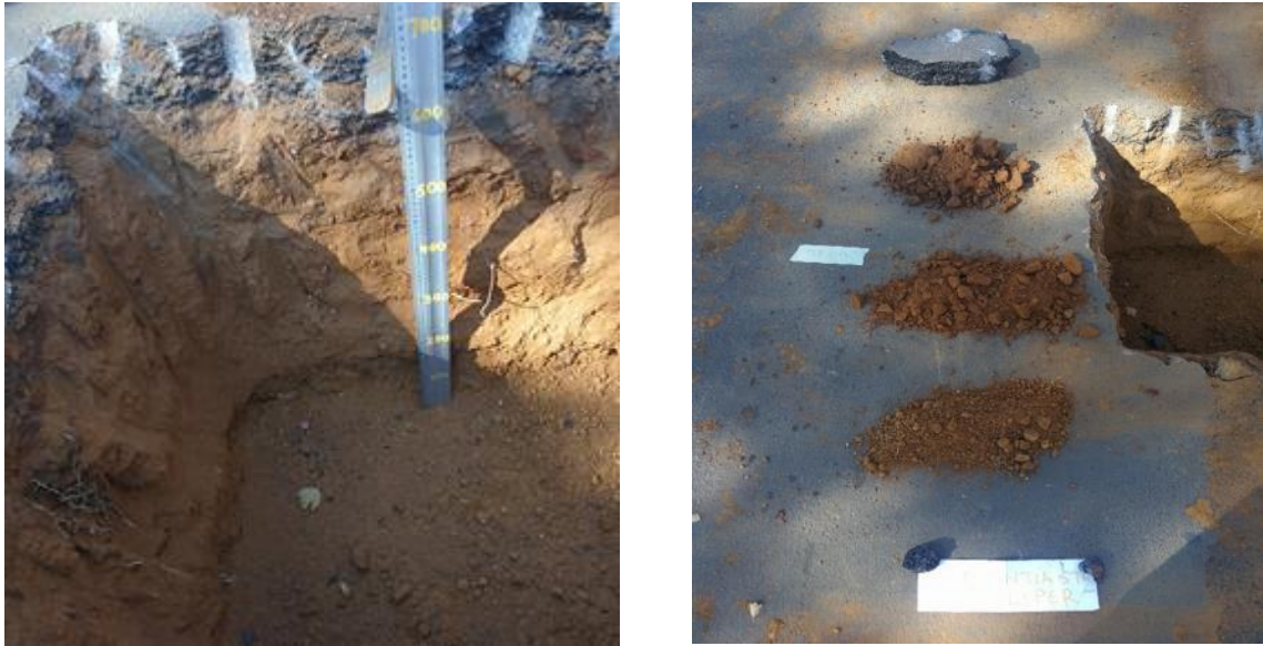
Photo 31: Test Pit 4 profile and pavement materials
