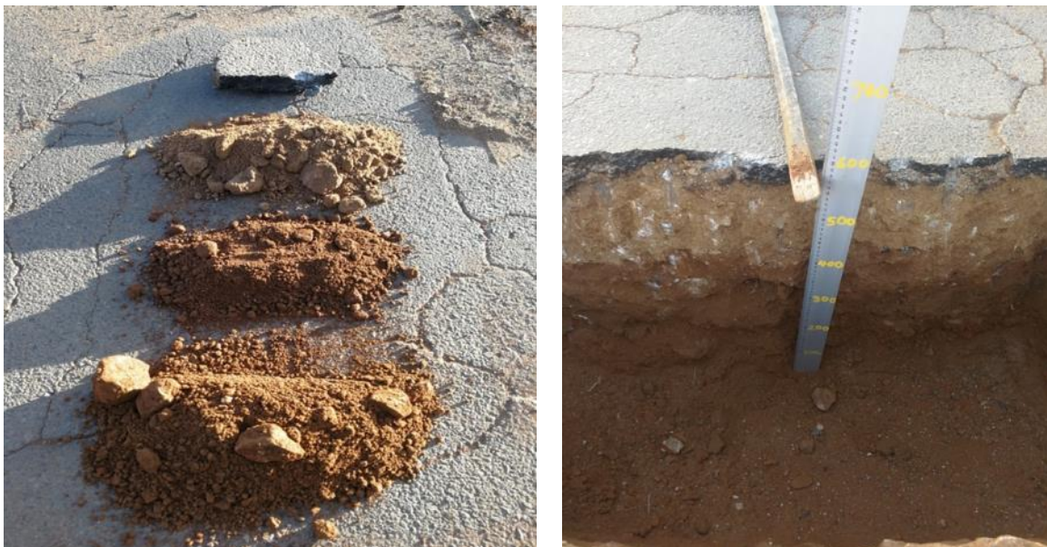
Photo 29: Pavement materials: Test Pit 2 between Maple Street and EP Malan Street
