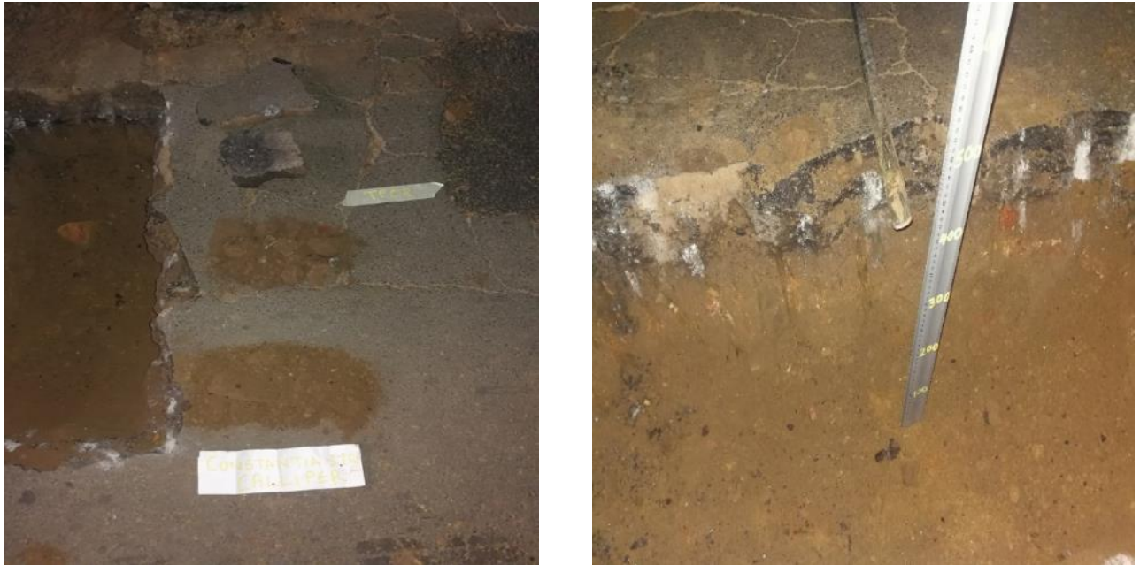
Photo 30: Pavement materials: Test Pit 3 between EP Malan Street and Elgin Street
