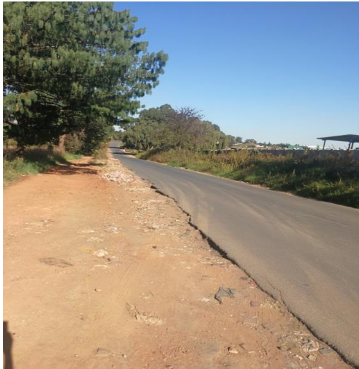
Photo 22: Road prism between EP Malan Street and Elgin Street
