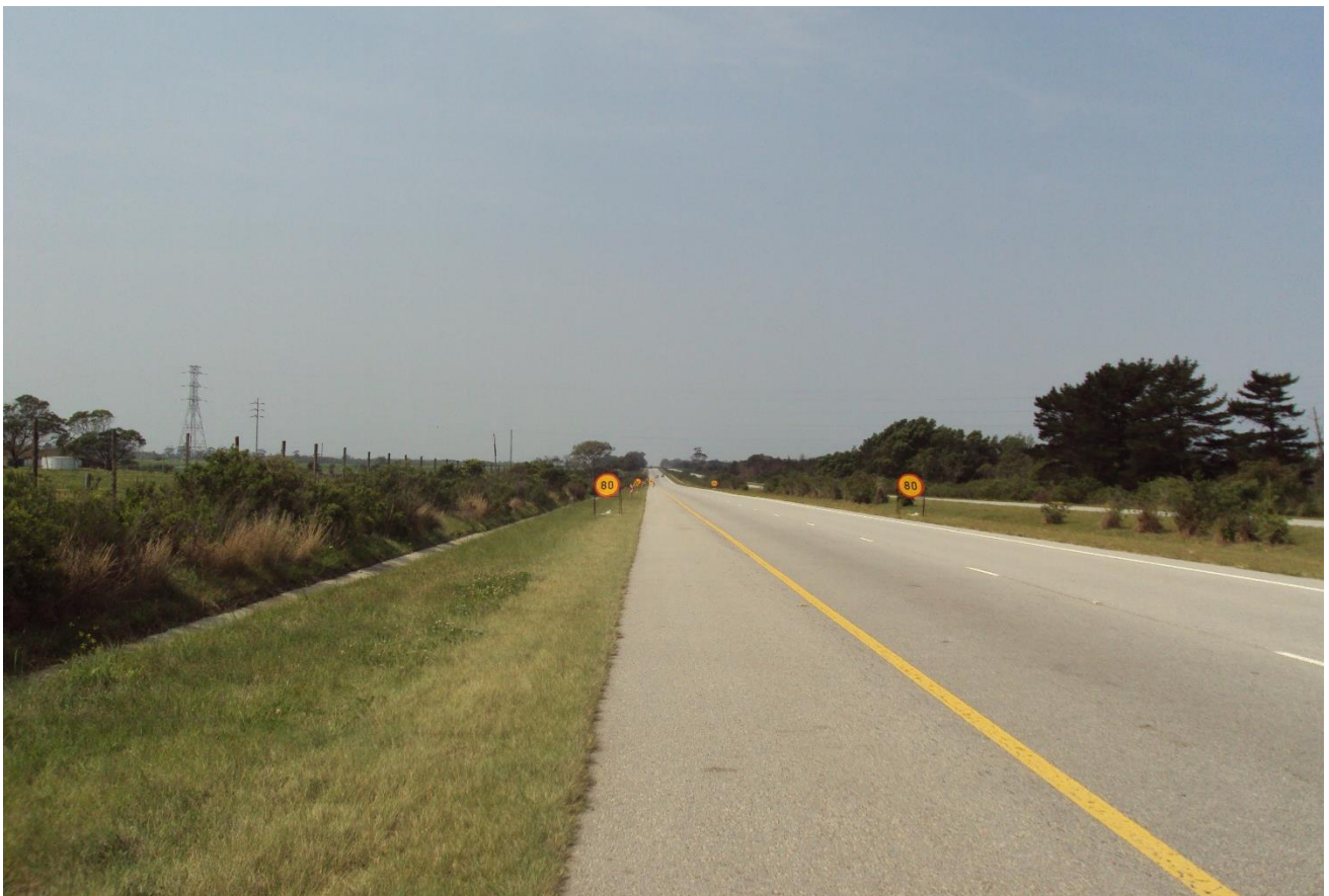
Figure 50: Existing Eskom 132kV overhead powerline visible from the N2
