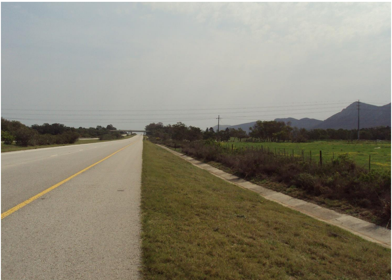
Figure 52: Existing Eskom 132kV overhead powerline crossing the N2 near Lady's Slipper
