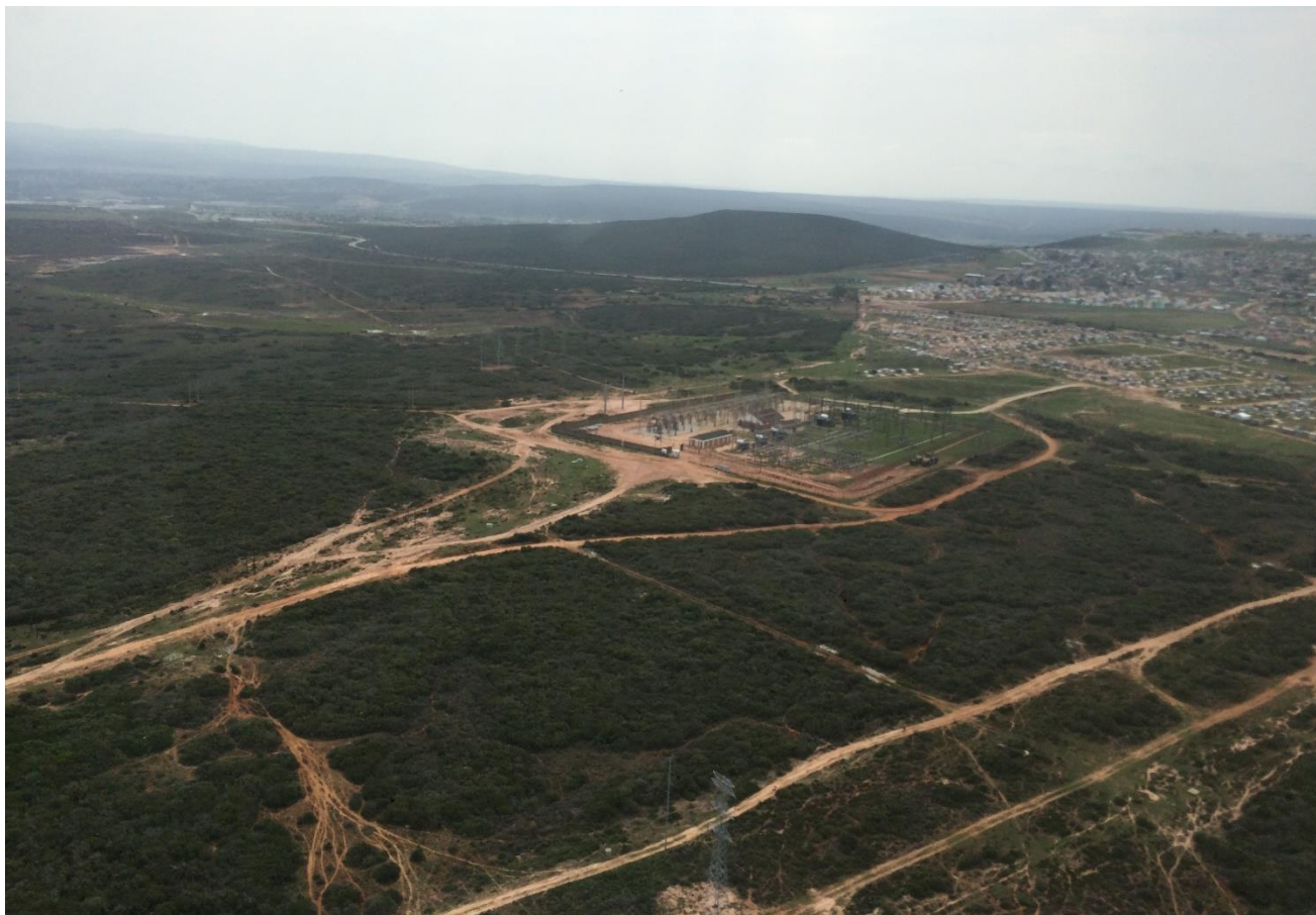
Figure 53: Aerial photograph of Sans souci substation on the outskirts of the urban edge (source: Palmer, 2017)
