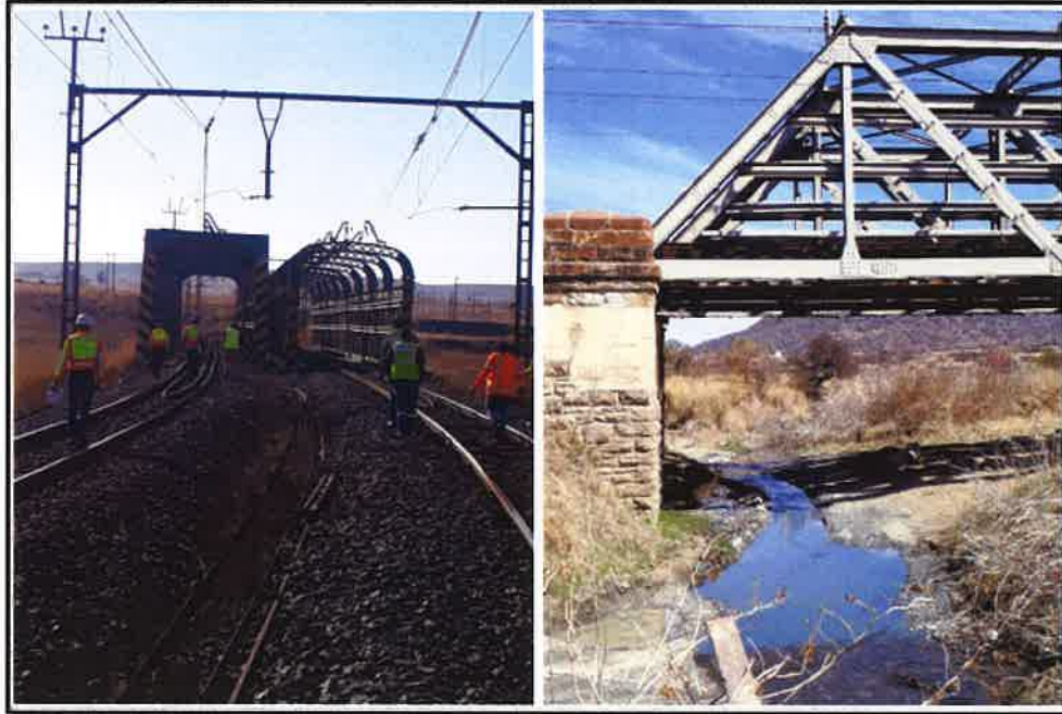
Figure 4: Example of the bridges where the OHTE work will be done
