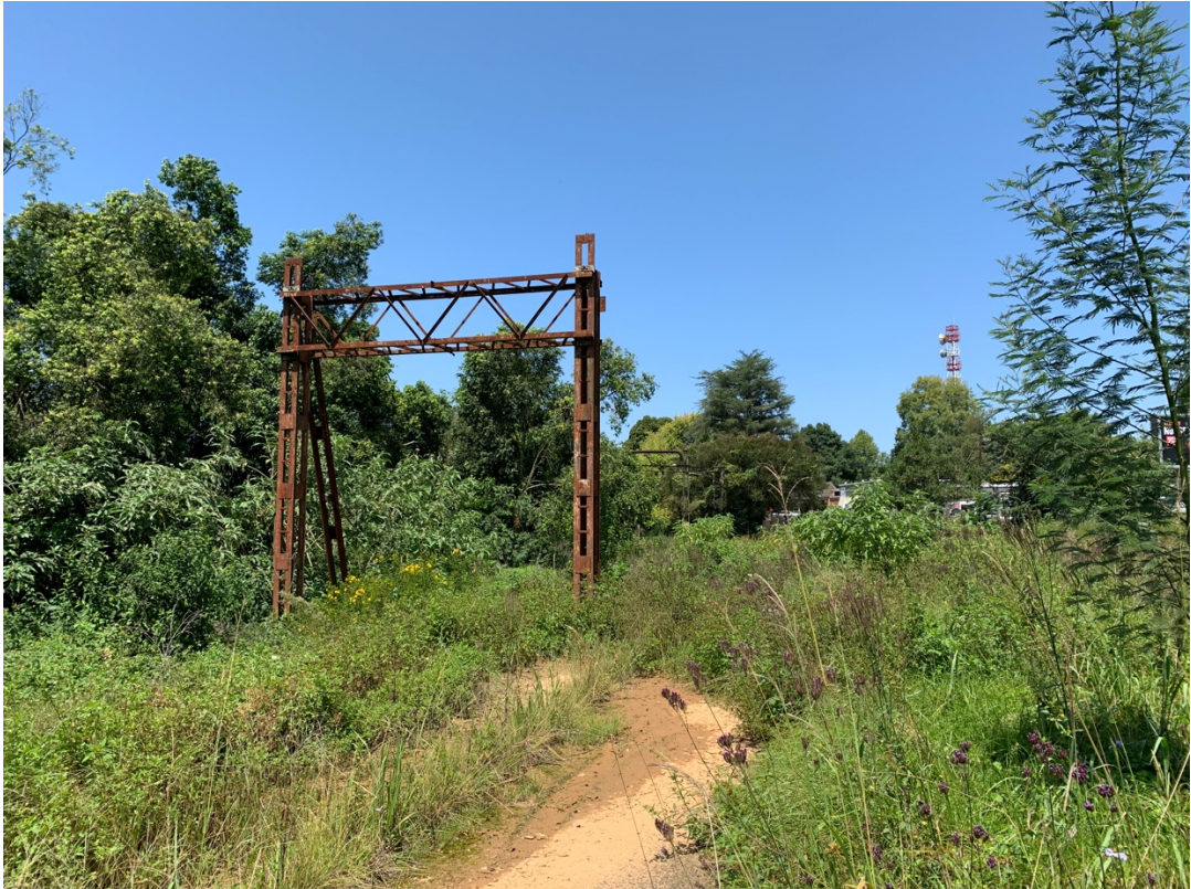
7- The steel gantry on the southern end of the site
