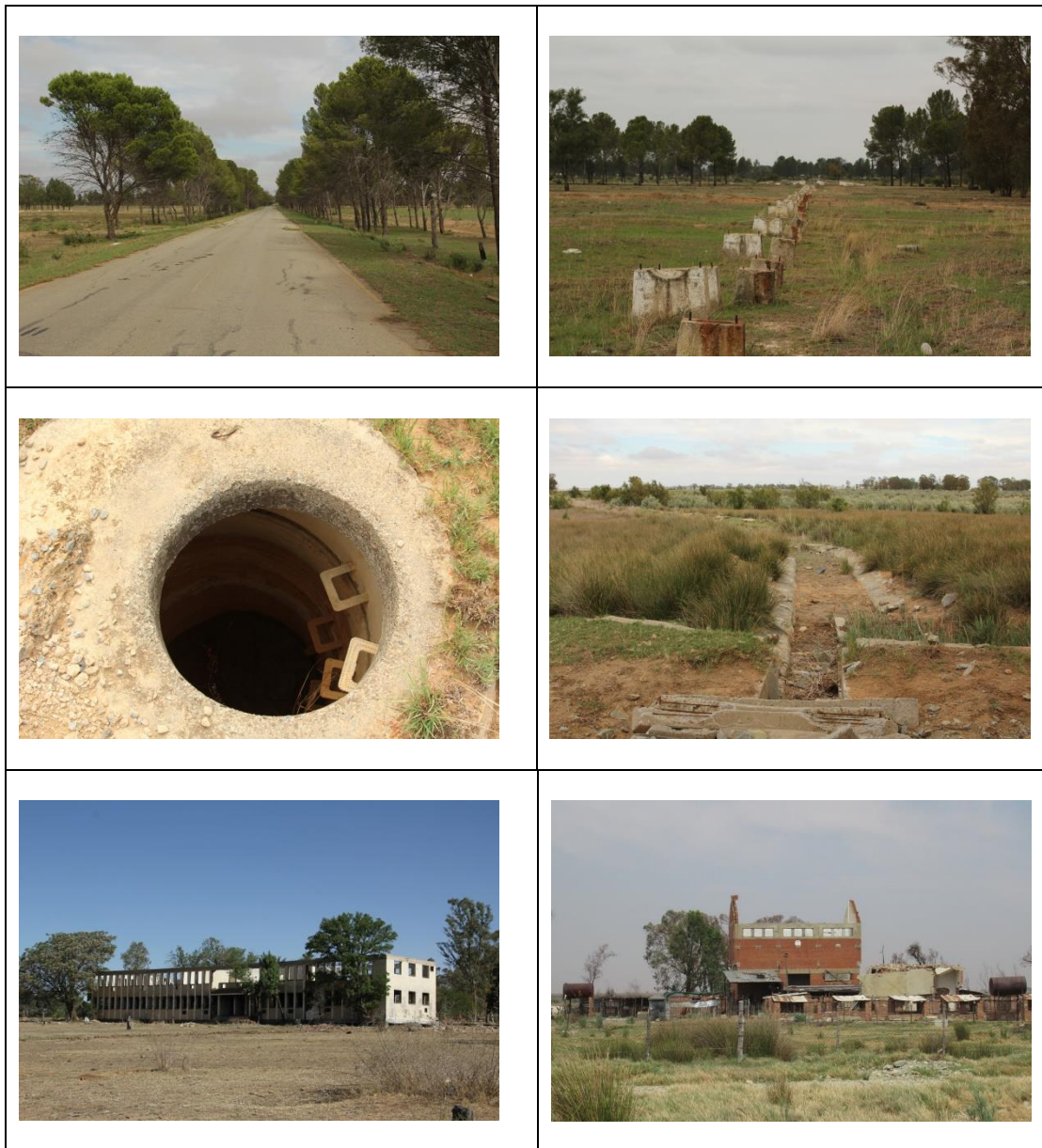
Figure 4. The remains of mining related infrastructure.
