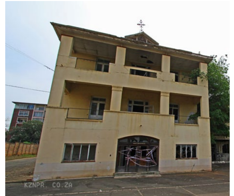
BLOCK A / EXTERIOR
