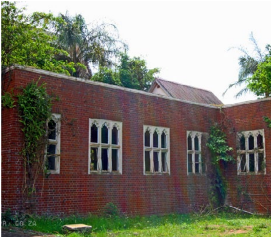
BLOCK E / CHAPEL / EXTERIOR
