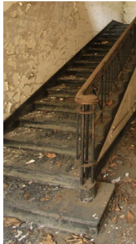
BLOCK C / STAIRCASE
