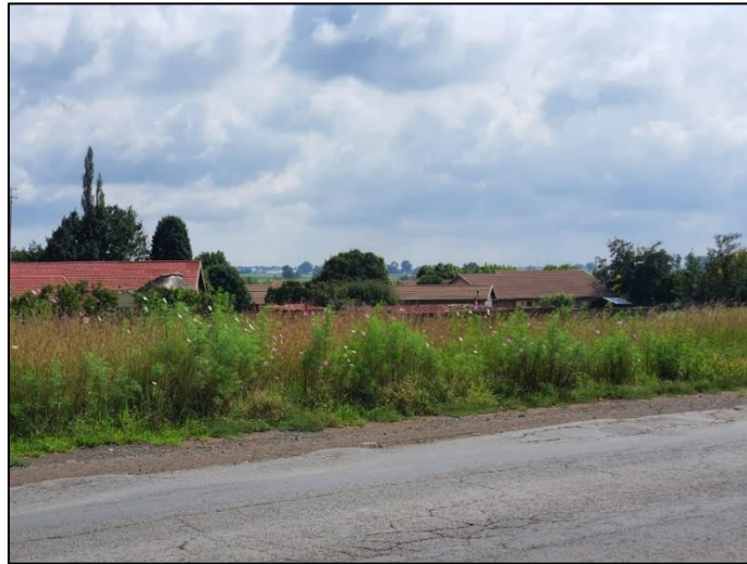
Figure 3-7: View of the proposed alignment for the preferred pipeline route along the R39 road in Standerton.
