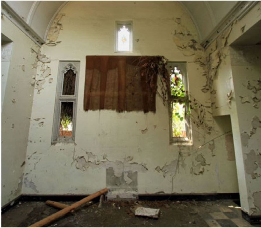
BLOCK E / CHAPEL / INTERIOR
