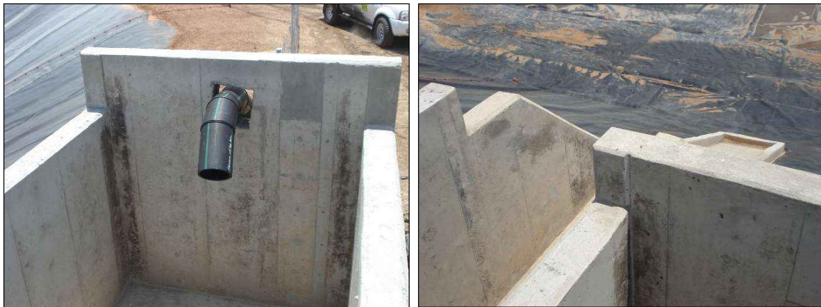
Figure 8-1, 8-2 & 8-3 : Typical Pump Inlet Structure with Silt Trap
