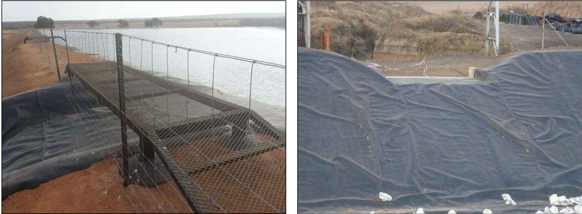
Figures 5-1 & 5-2 : Typical Emergency Spillways
