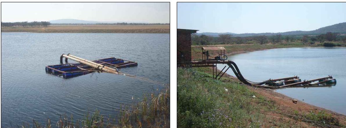
Figures 6-1 & 6-2 : Typical Suction Pipes with Floating Structures
