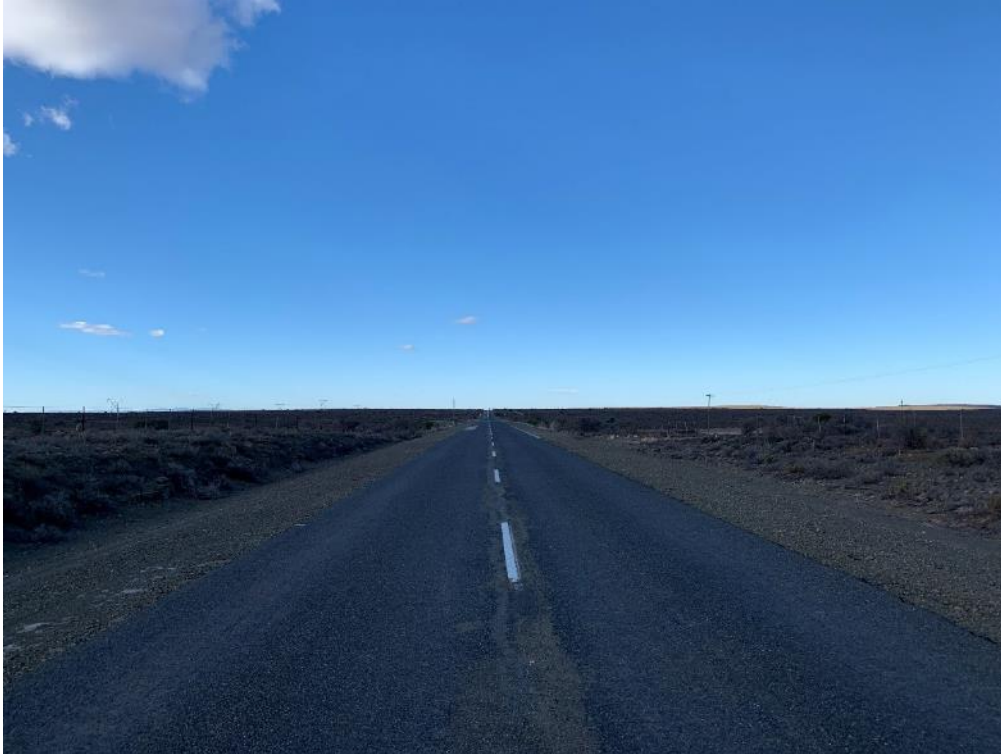
Figure 7.5 Existing Portion 10 Access – North approaching
