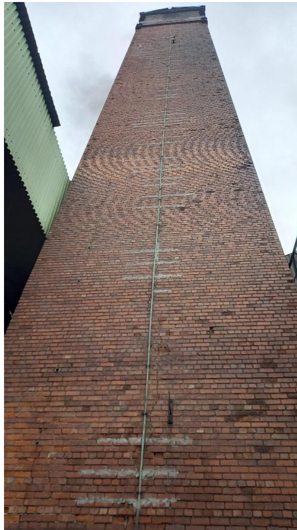
Existing Boiler Stack to be replaced
