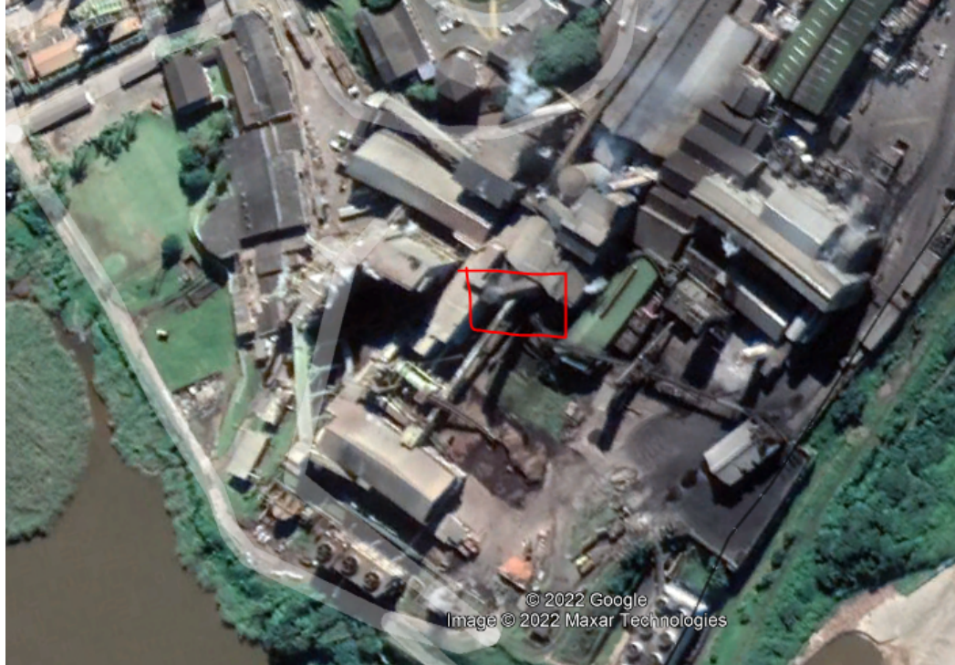
Google Earth Imagery of the Plant in Sezela with the location of the existing stack in red
