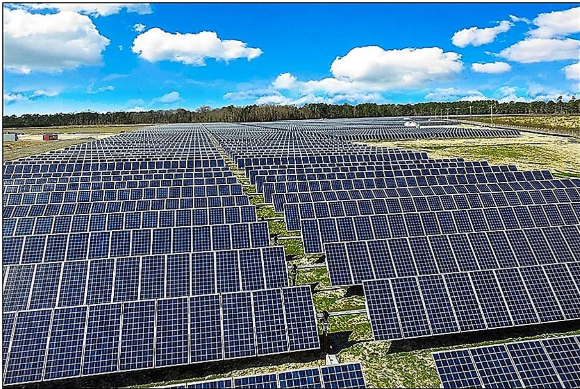
Figure 2.1: Typical example of solar PV array
