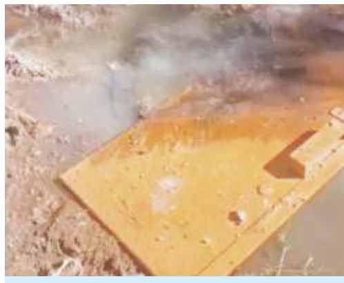
The overflowing sewage manhole.
