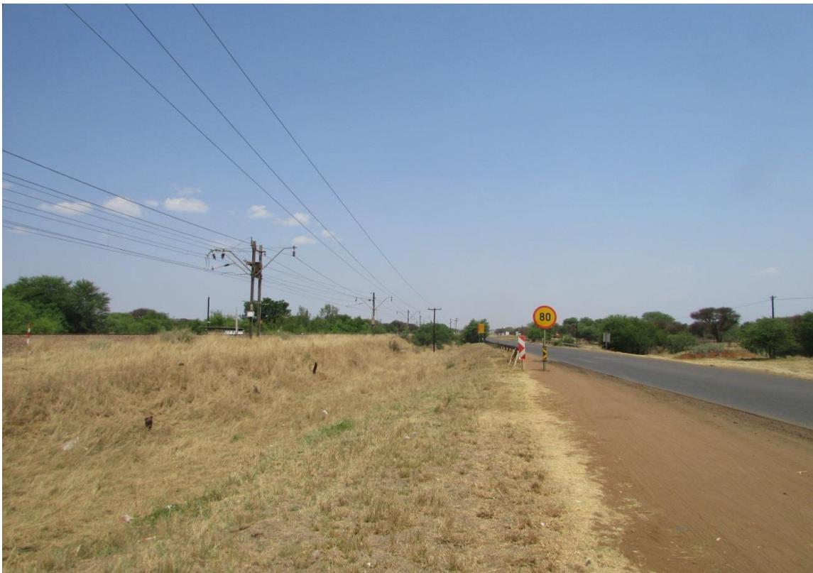
Figure 19: A view of a section of the line route running between Northam (along the R510) up the connection with the new transmission line close to Bojating Village and the PV Facility. Note the railway line as well.
