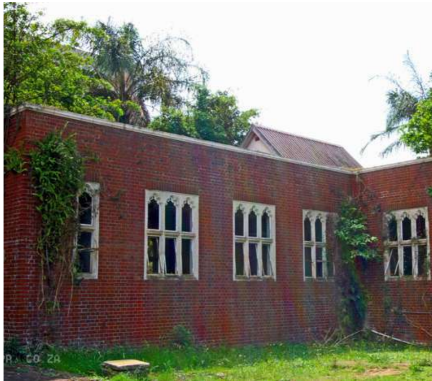
BLOCK E / CHAPEL / EXTERIOR
