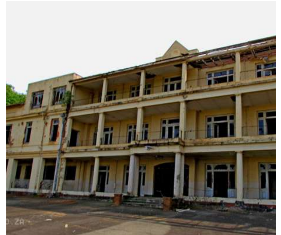
BLOCK F / EXTERIOR
