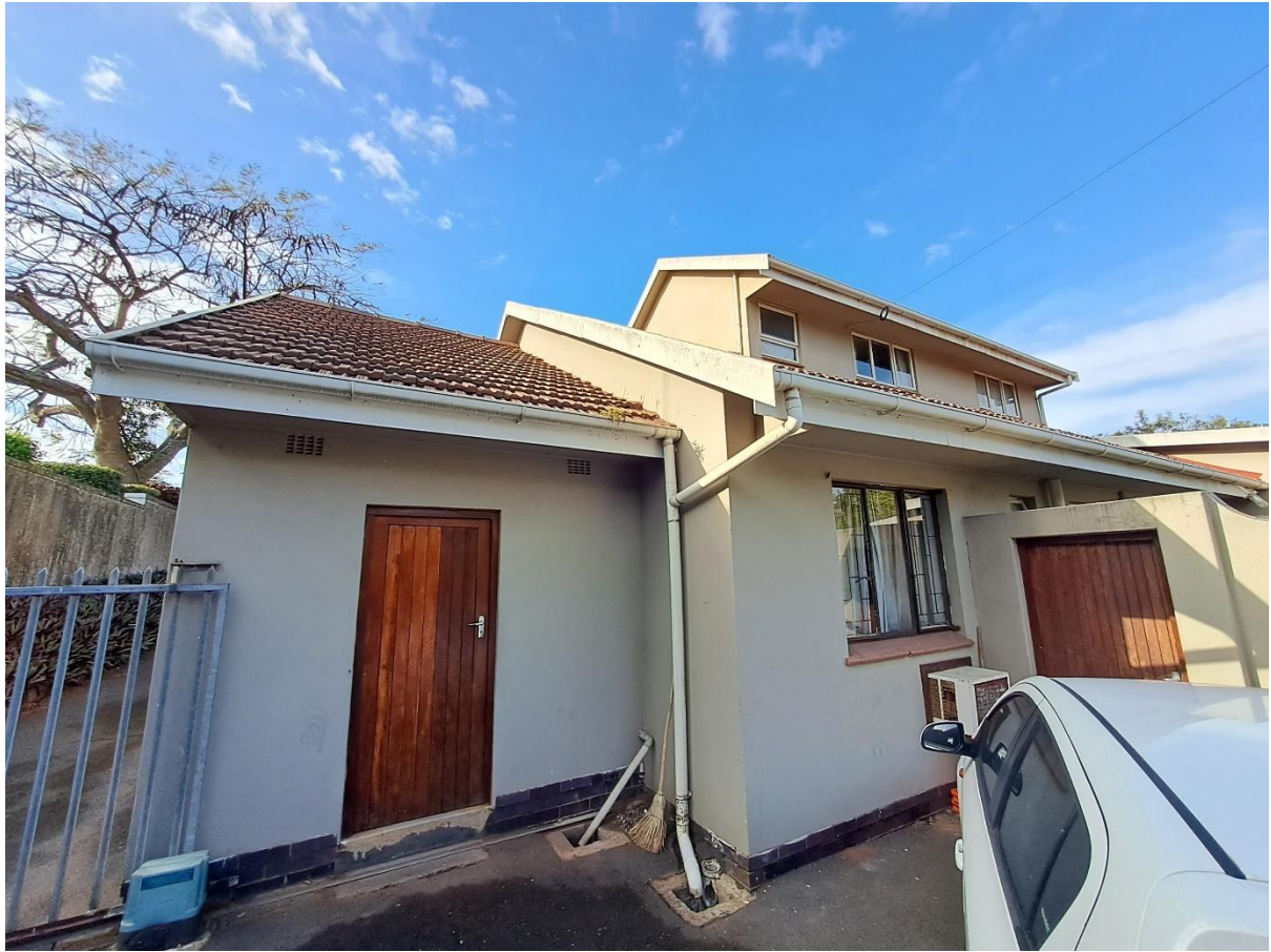
The existing laundry room.
