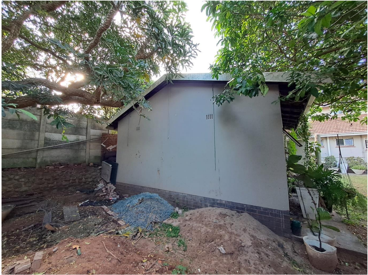
The existing garage's back of the building.
