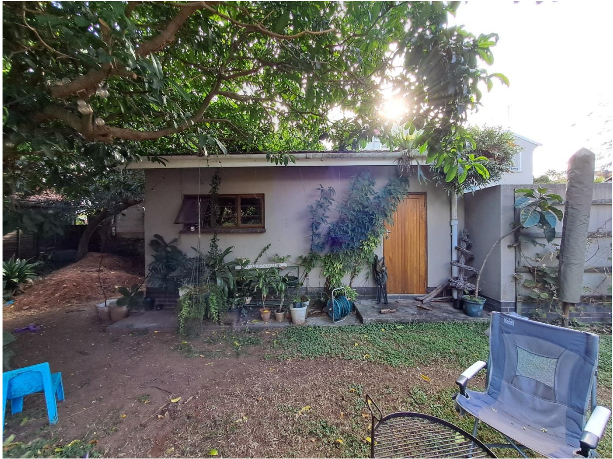
The existing garage.
