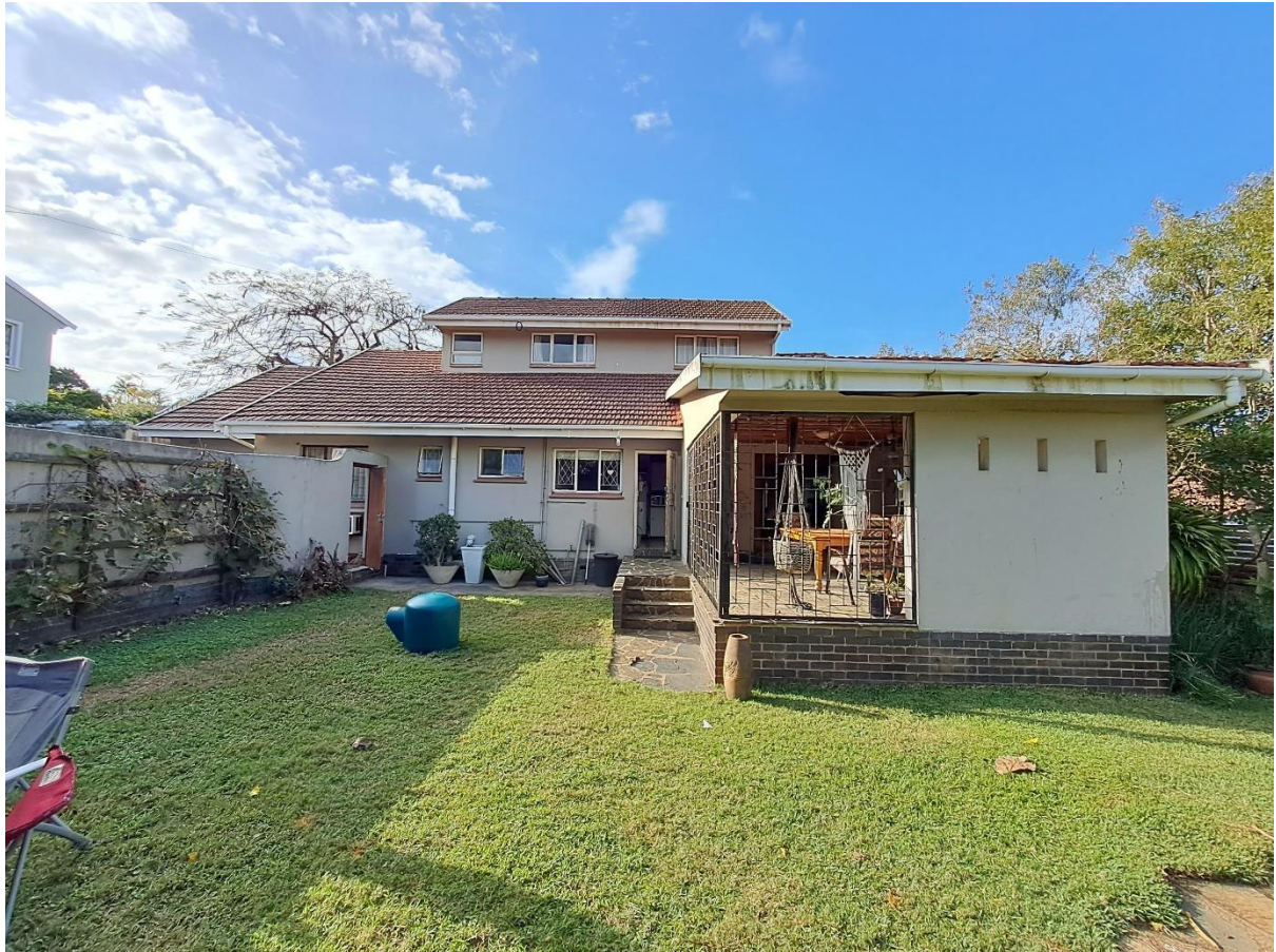
The existing verandah that will be extended.
