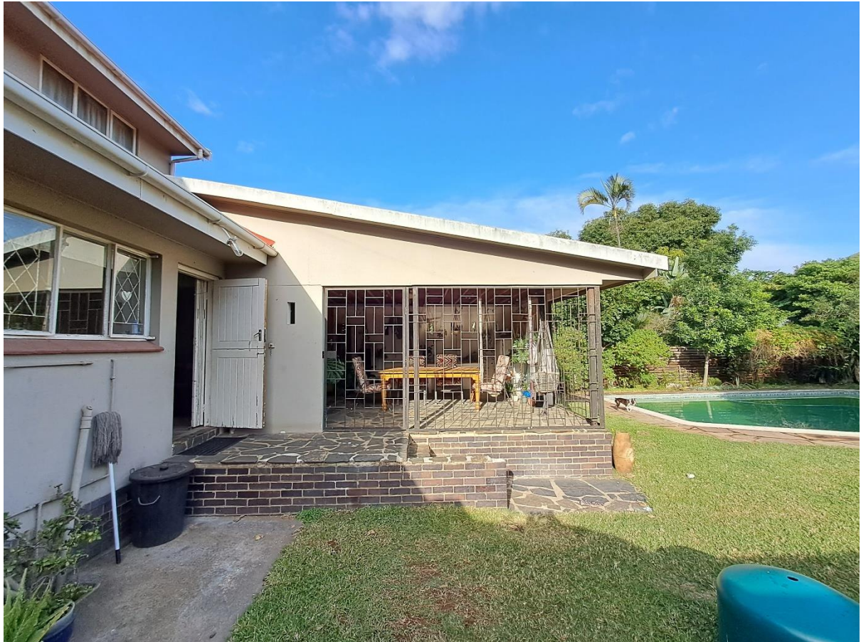
The existing verandah that will be extended.
