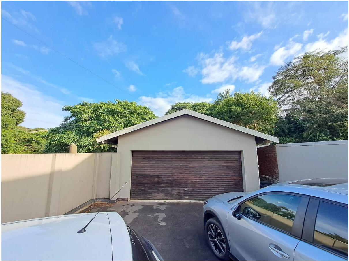
The existing garage door.
