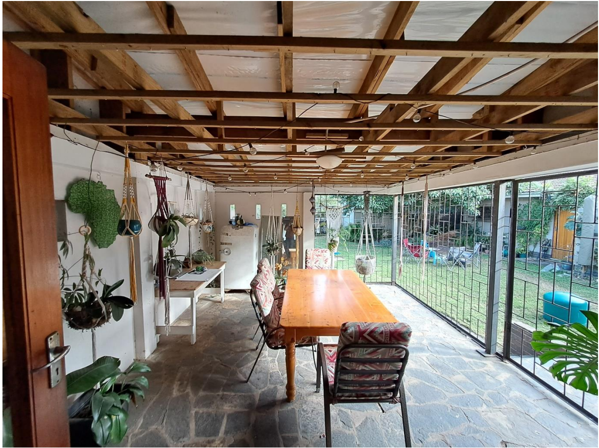
The existing verandah that will be extended.
